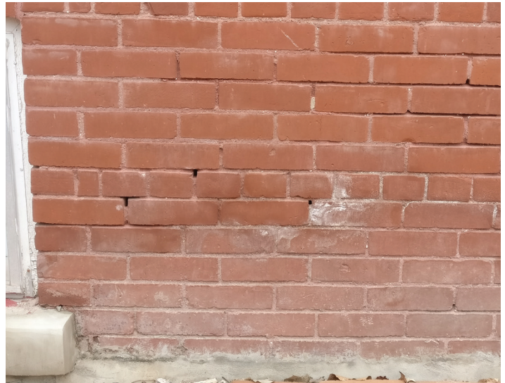
Missing and Degraded Mortar
