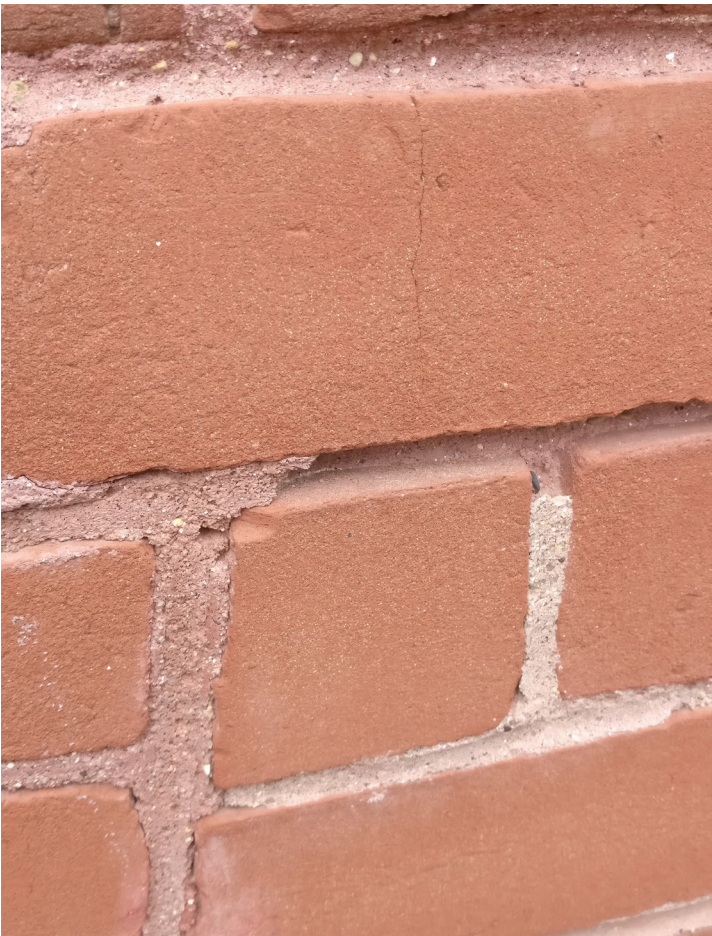
Repointing with Different Mortar Types
