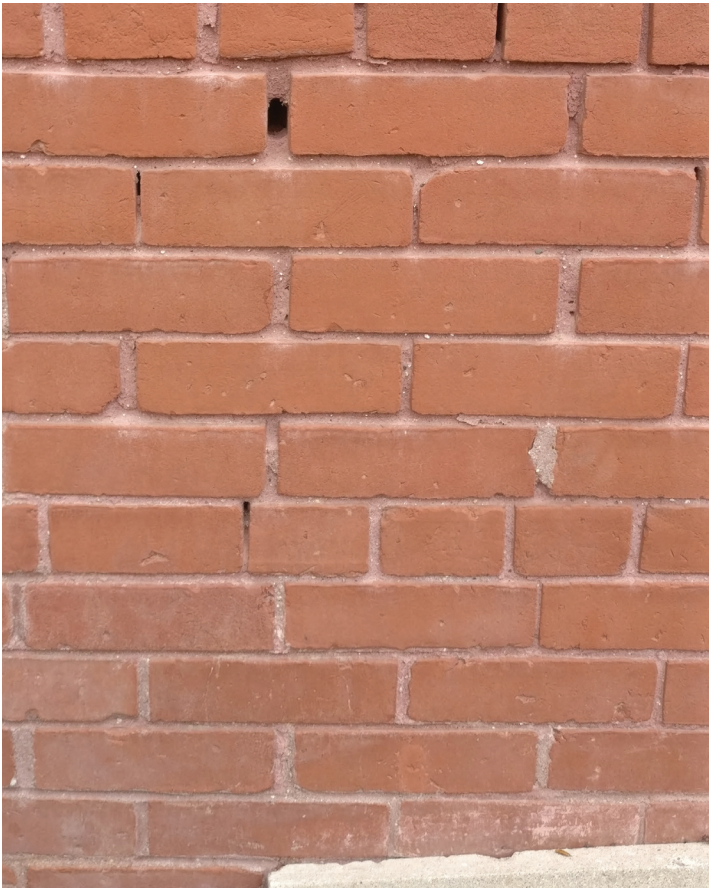
Repointing with Different Mortar Types and Missing Joints
