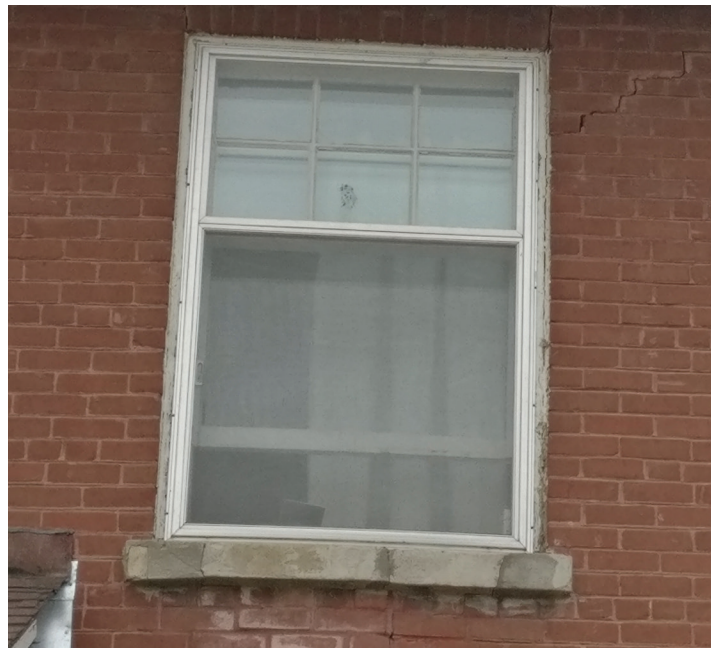
Original Second Floor Window with New Storm Window
