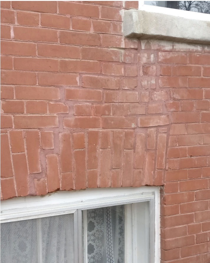
Incorrect Brick Repair South Facade
