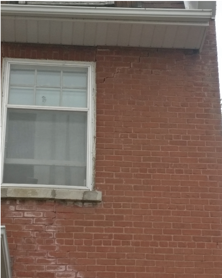
Mortar Patching and Pushed Face Brick South Facade
