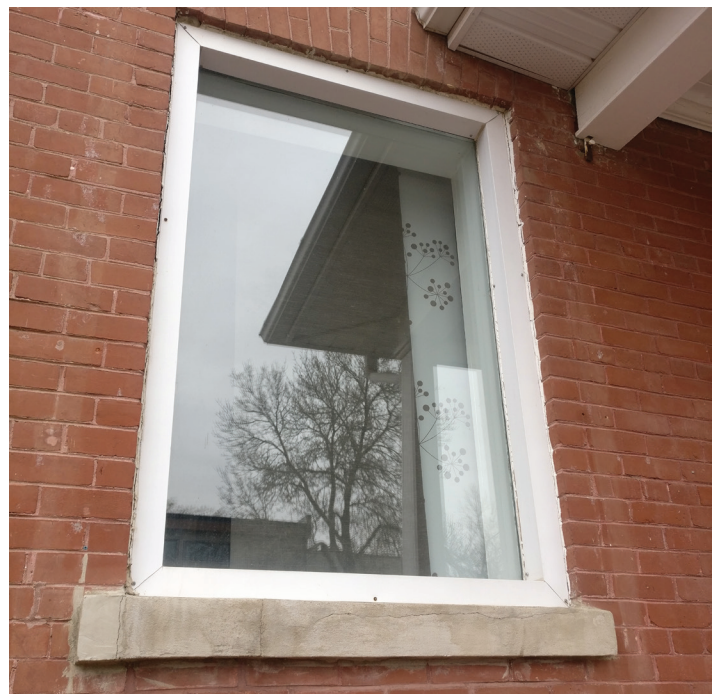
Missing Stucco on Sills
