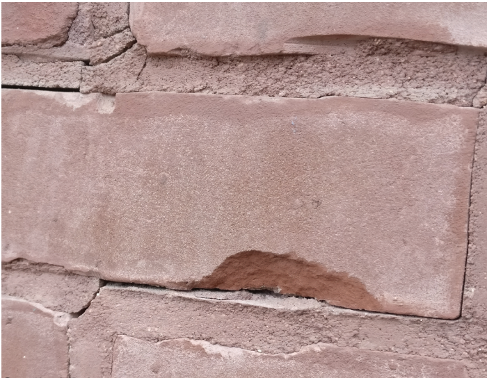
Spalled Brick
