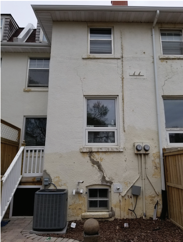
Stucco Cracking and Patching North Facade
