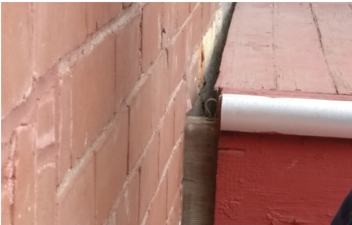
Separation of Porch From Facade
