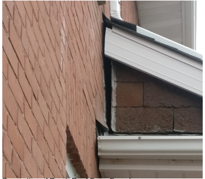
Separation of Porch Roof From Facade
