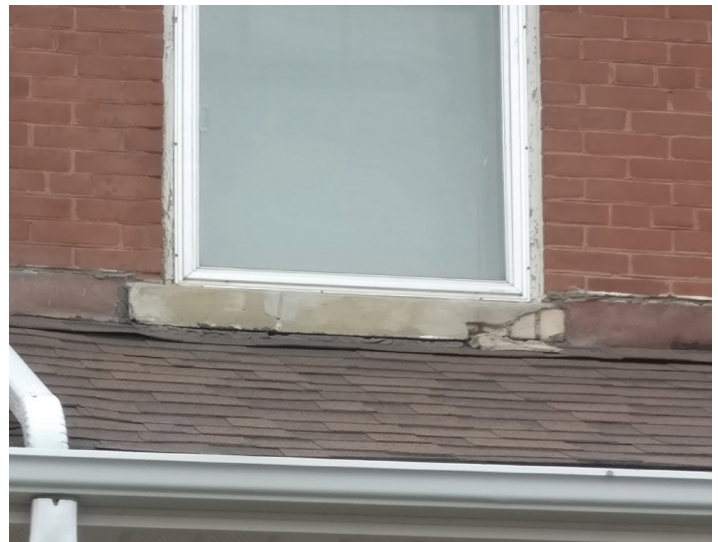
Missing Stucco on Sills
