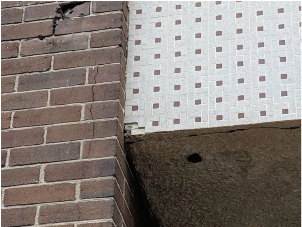
Photo 23: Cracked Brick and exterior tile
