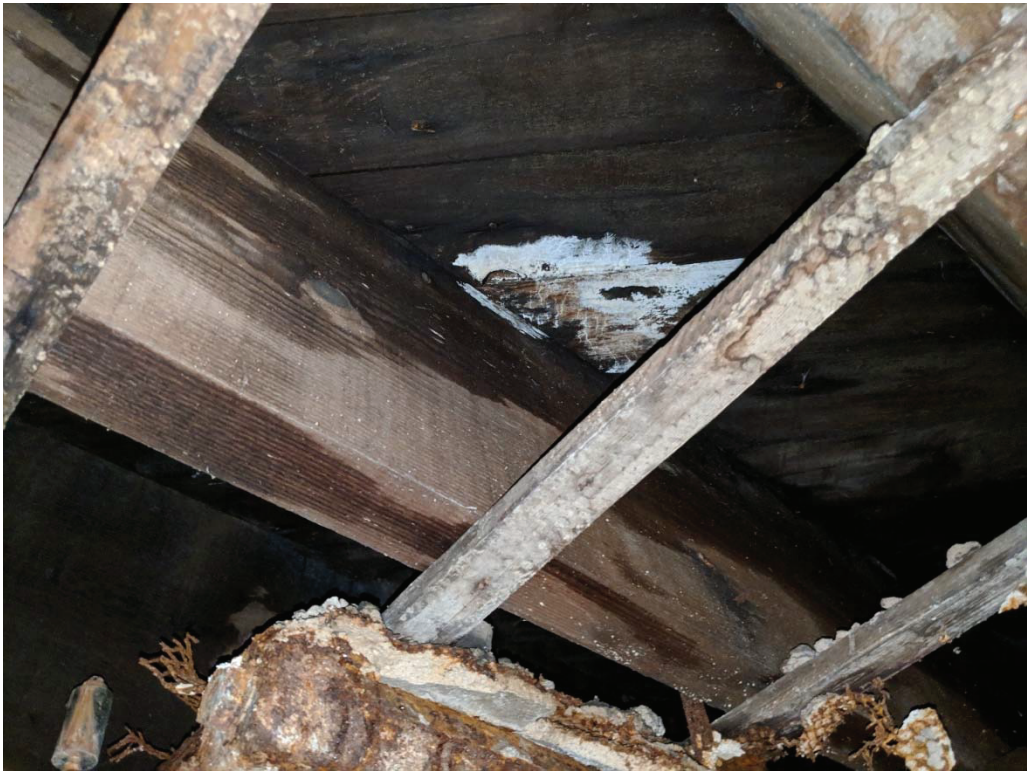
Photo 8: Rotting main floor wood decking and floor joist
