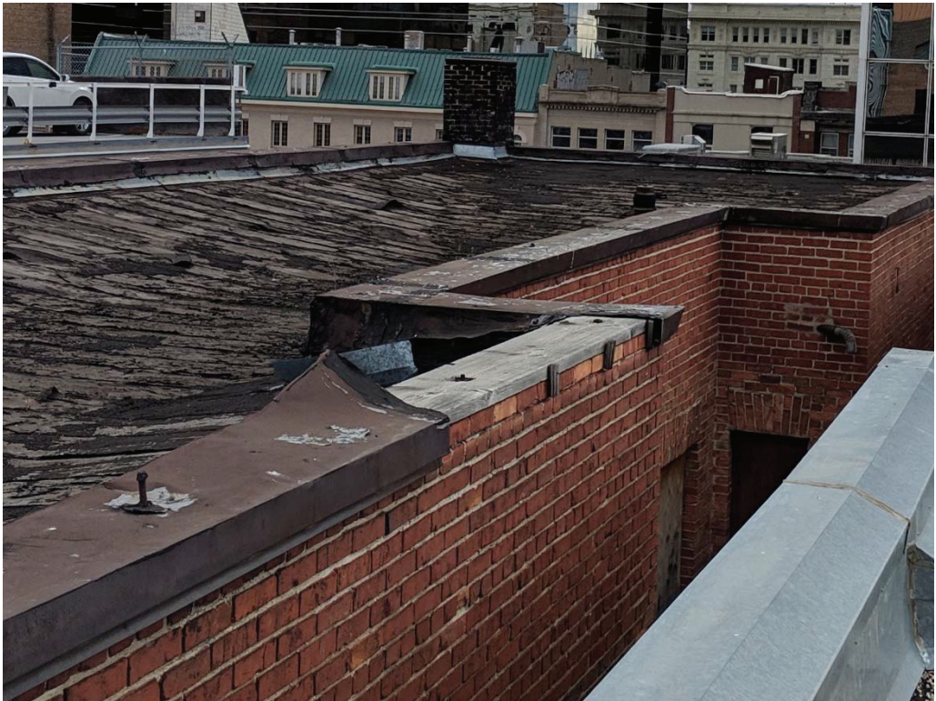
Photo 16: Missing parapet cap flashing
