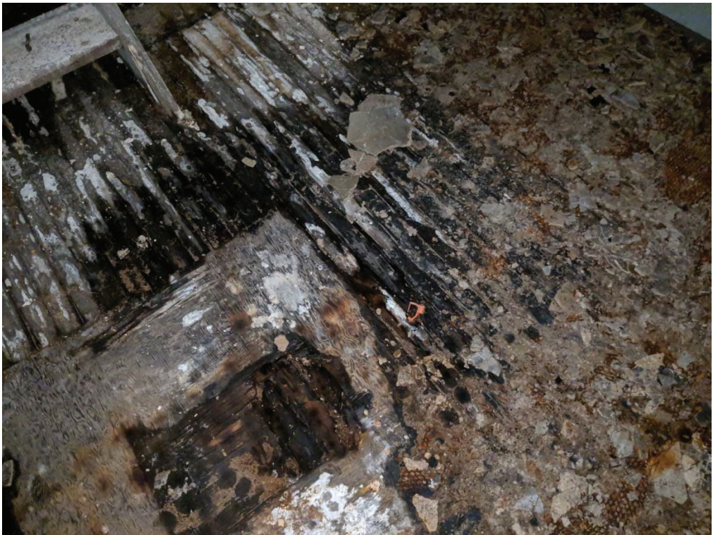
Photo 9: Rotting basement floor planks
