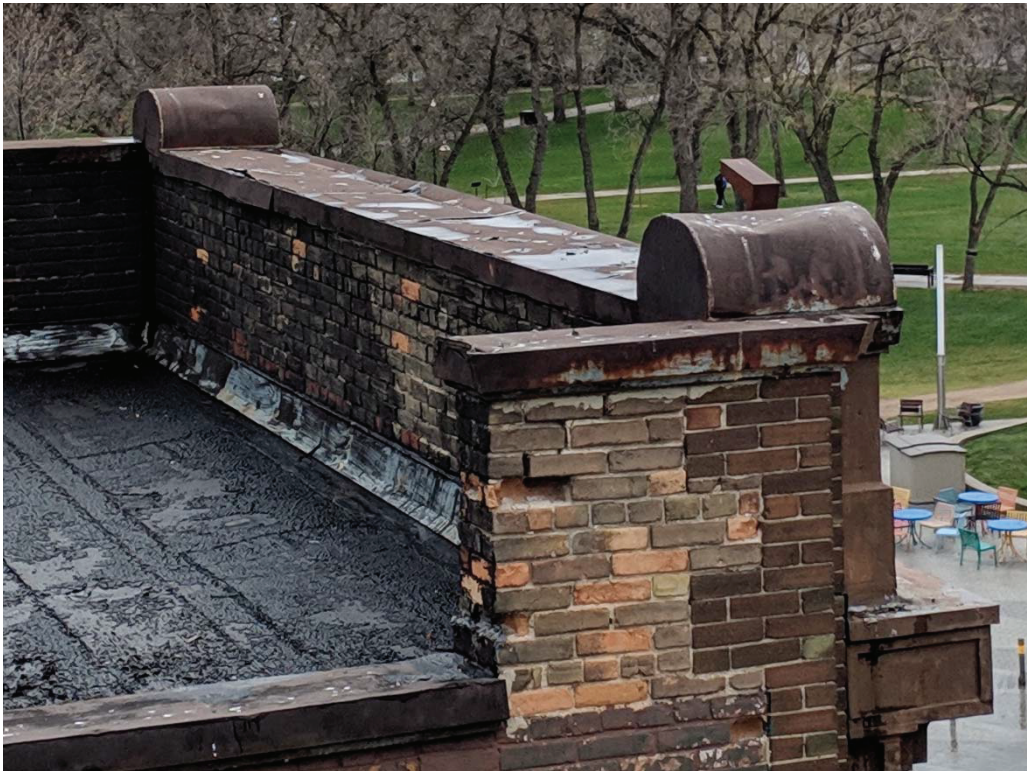
Photo 18: Damaged cap flashing over west parapet
