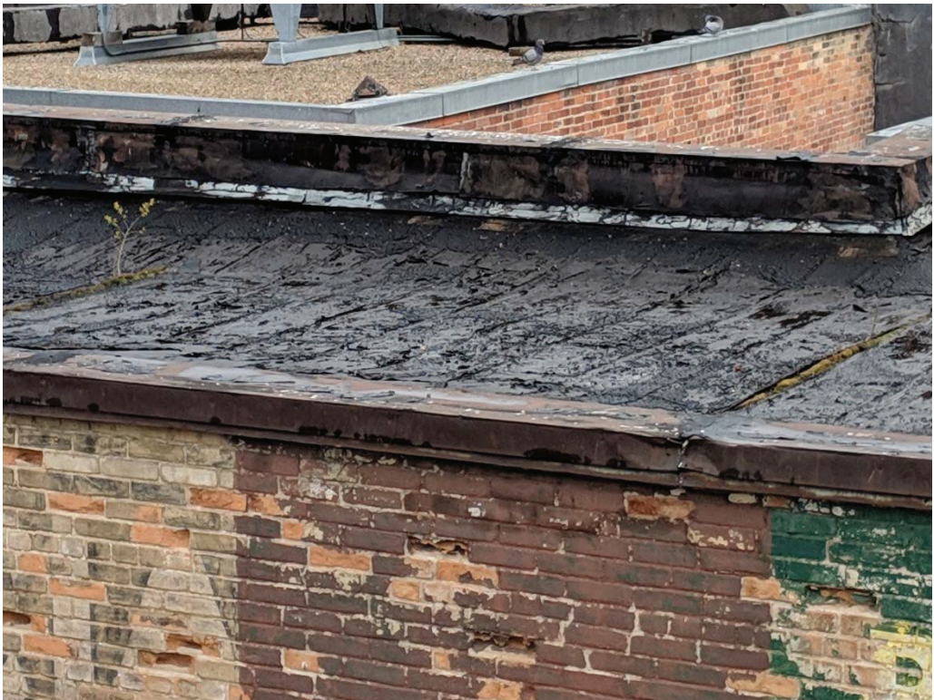
Photo 15: Deteriorated roofing and plant material growing on roof
