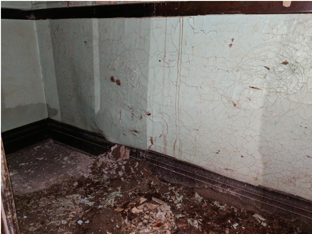
Photo 12: Cracked and deteriorated plaster walls
