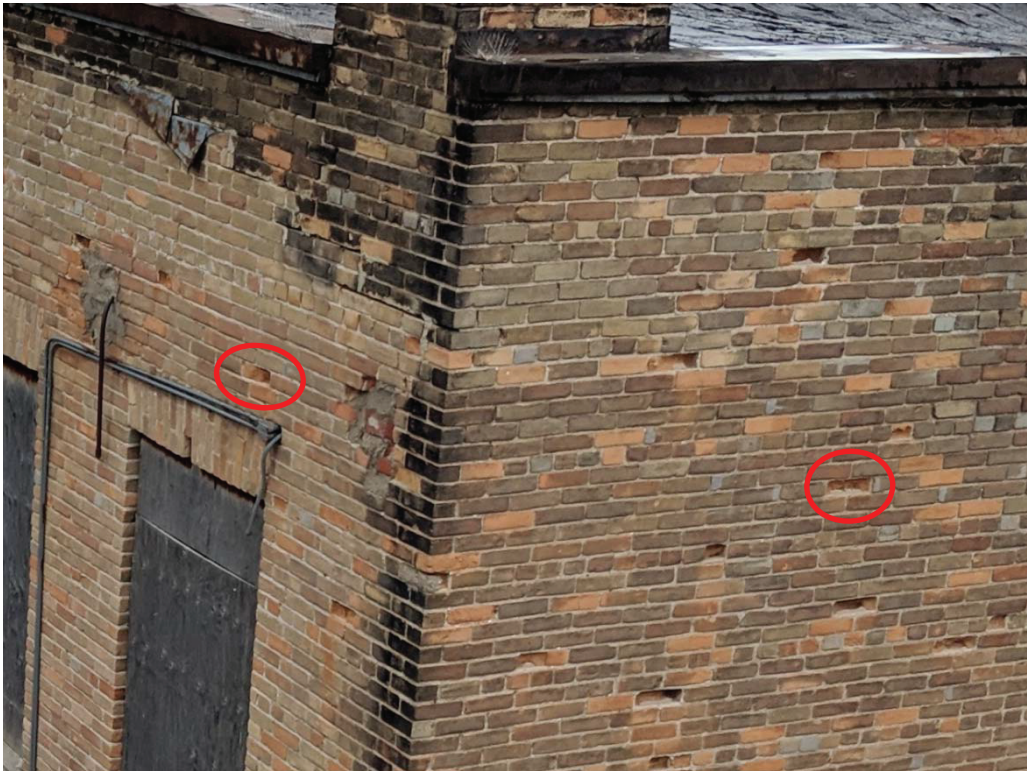
Photo 22: Spalled brick on north and east faces of building (Circled in red)
