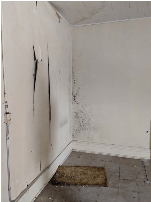
Photo 13: Potential black mold on second floor wall paper
