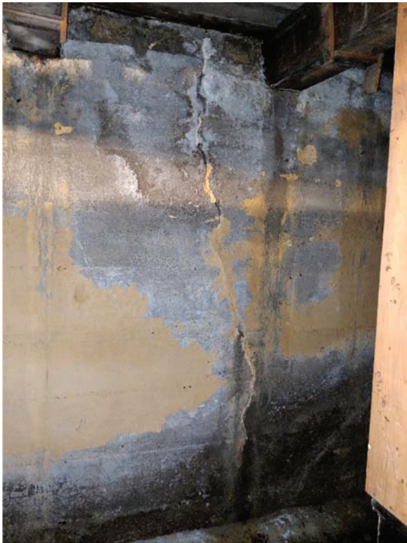
Photo 14: Crack in west foundation wall with efflorescence
