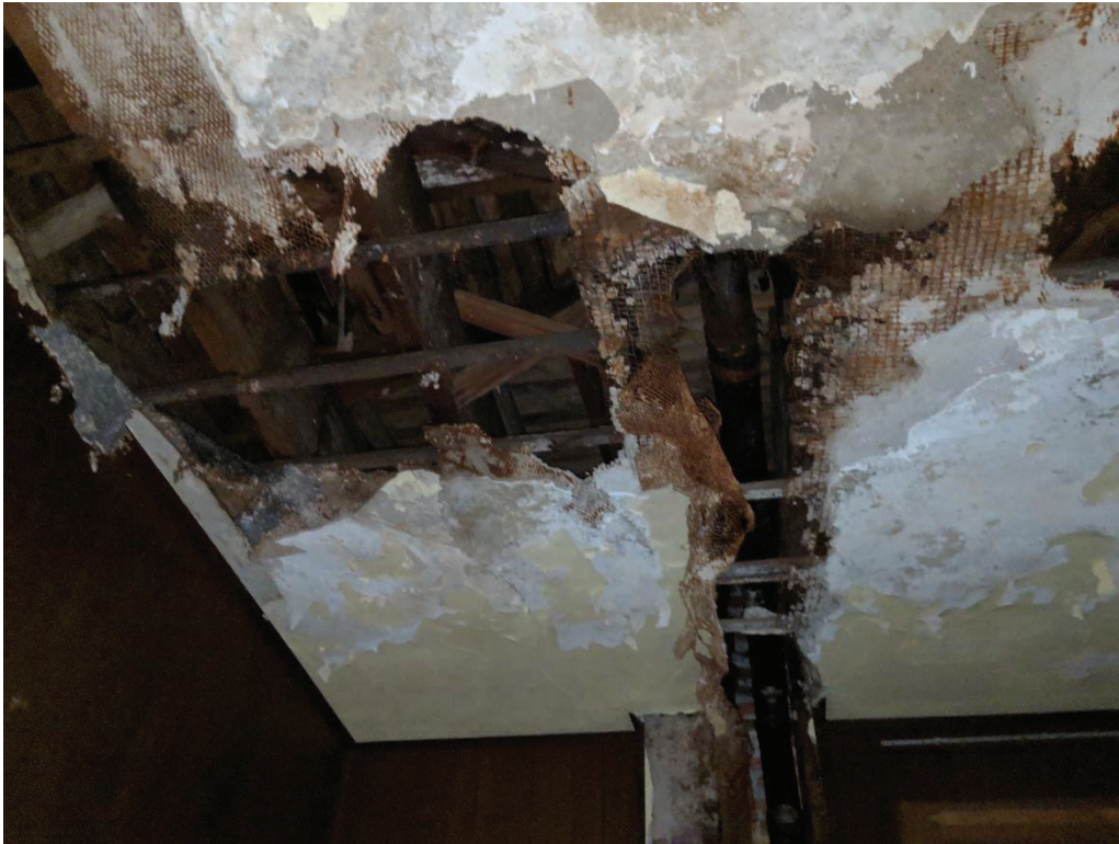
Photo 5: Third floor roof and steel mesh corrosion
