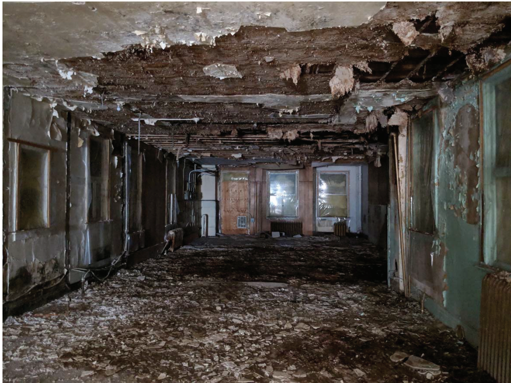
Photo 4: Second floor fallen ceiling
