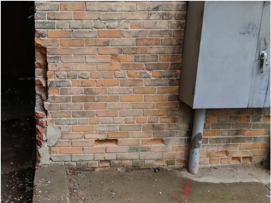
Photo 24: Spalled brick and hole in southeast corner of building
