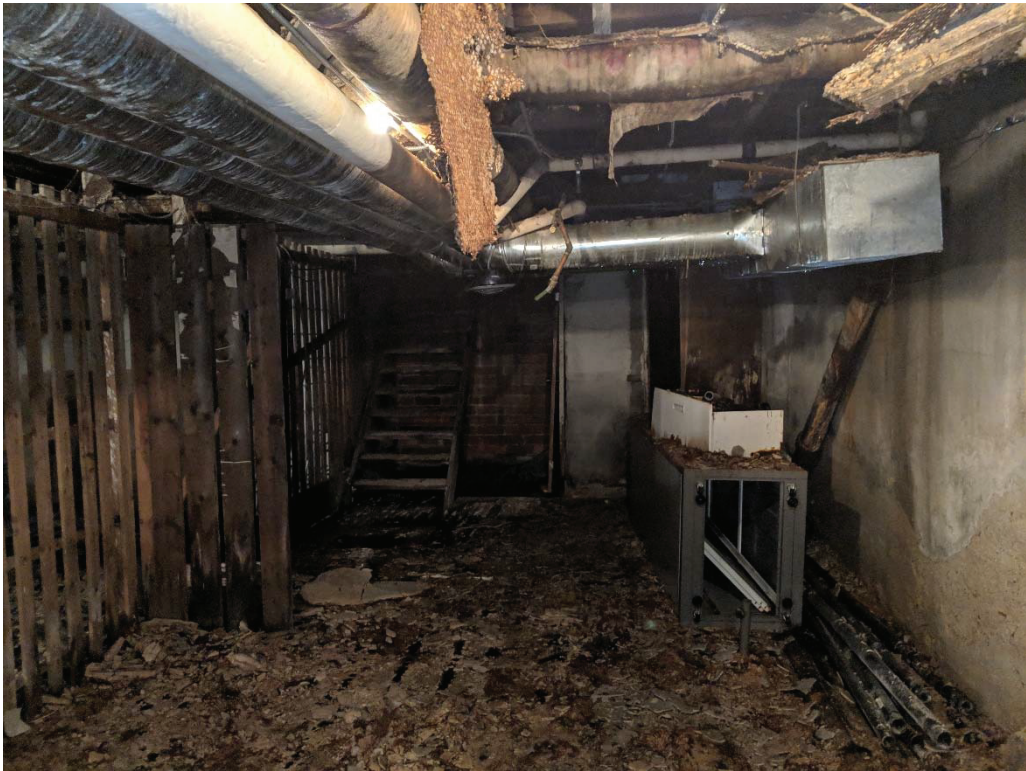
Photo 2: Basement fallen ceiling
