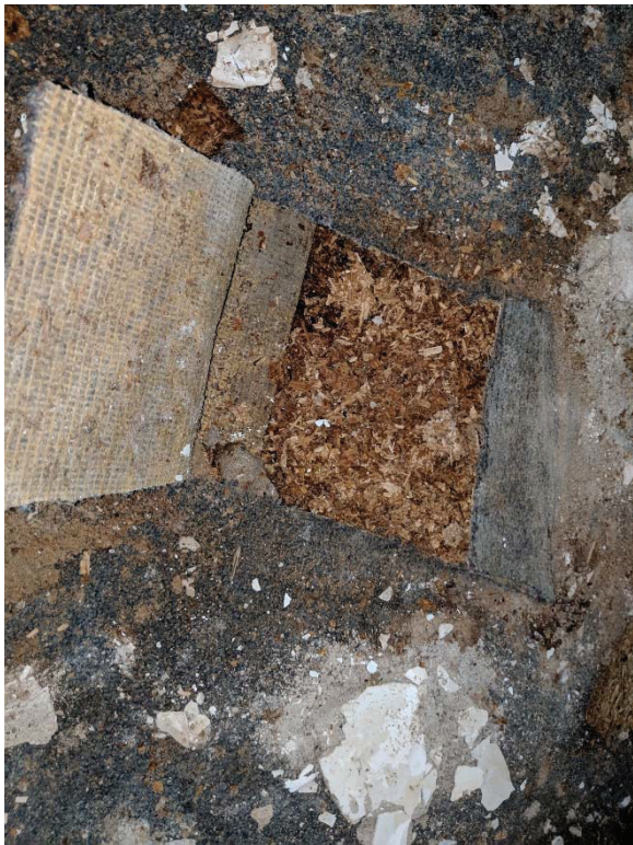
Photo 11: Wet and deteriorated chipboard sheathing on main floor
