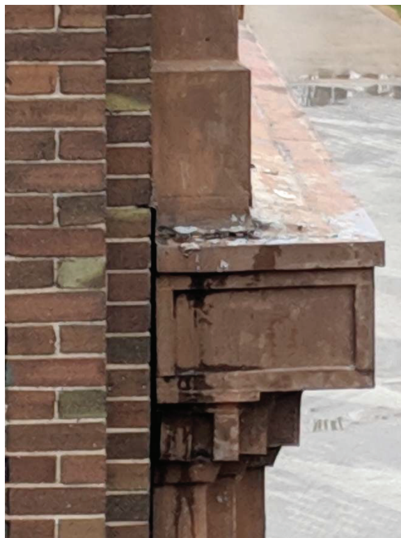
Photo 20: Deteriorated top edge of cornice
