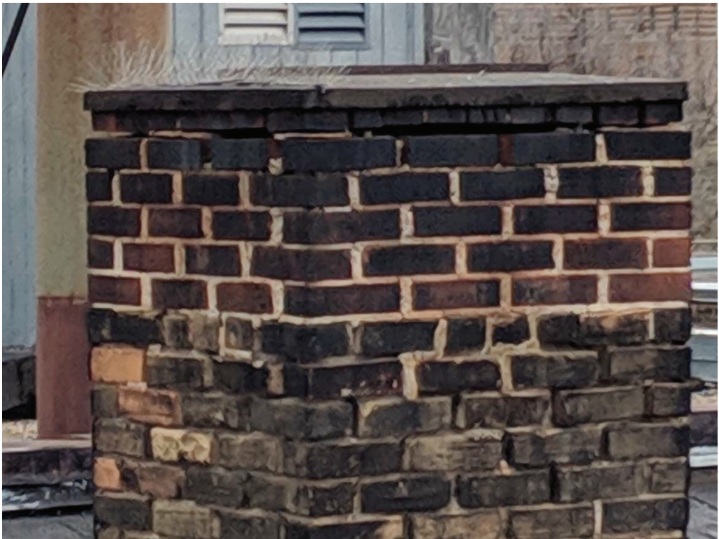
Photo 21: Deteriorated mortar on chimney
