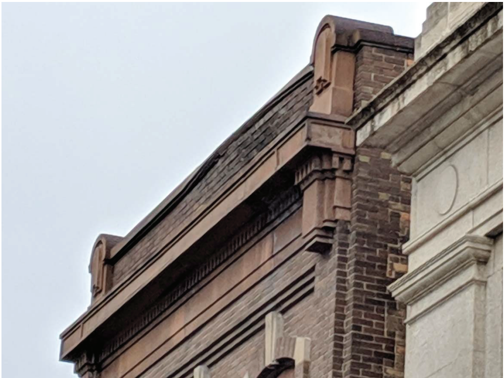
Photo 17: West parapet bowed outward
