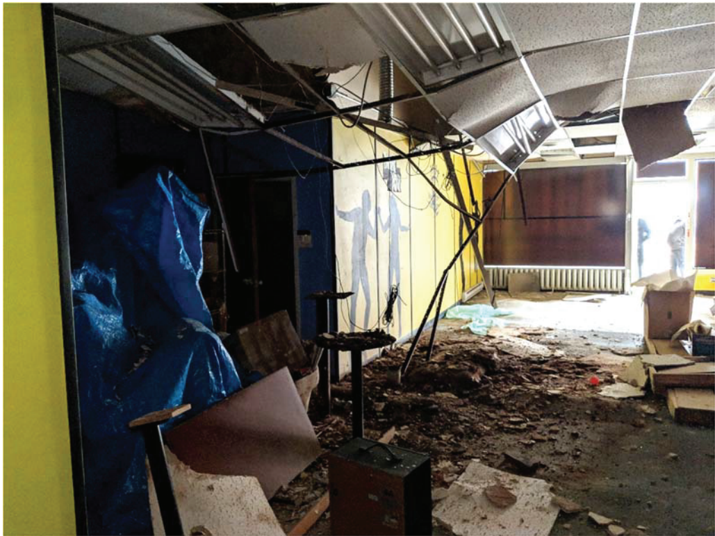
Photo 3: Main floor fallen ceiling
