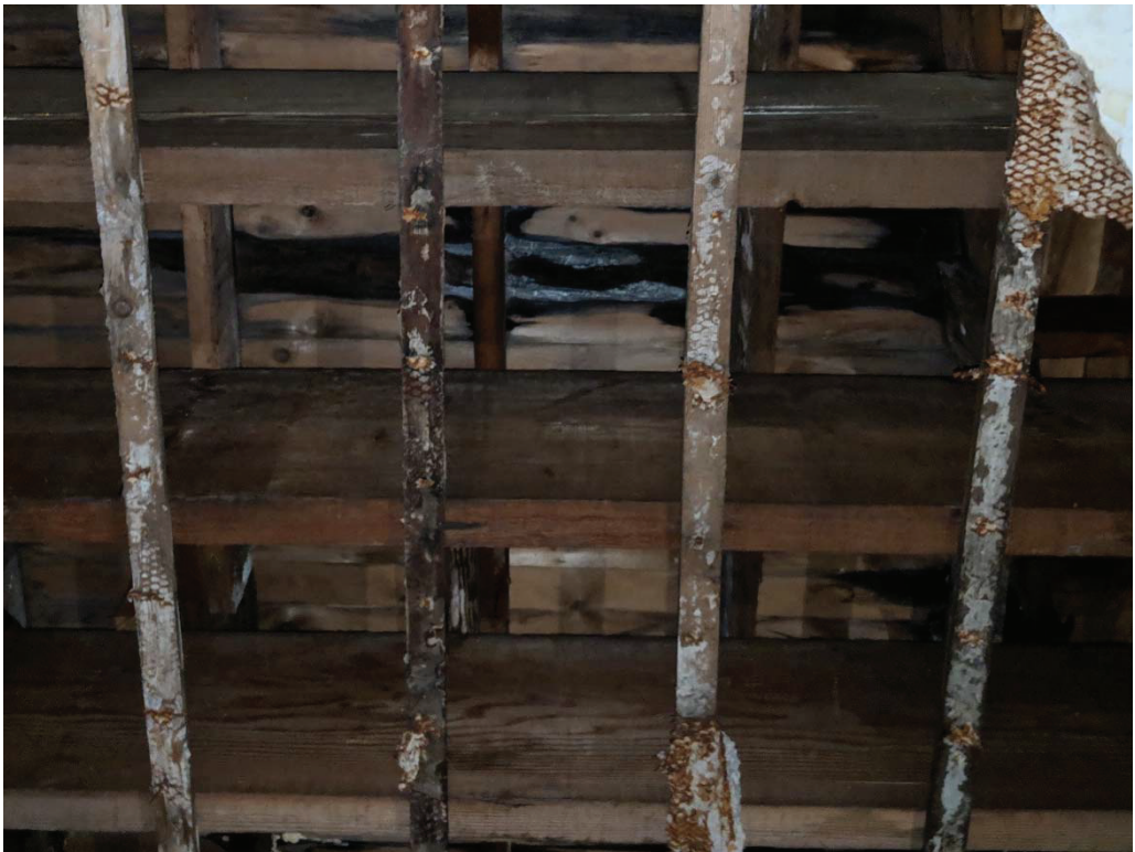
Photo 7: Rotting wood roof decking
