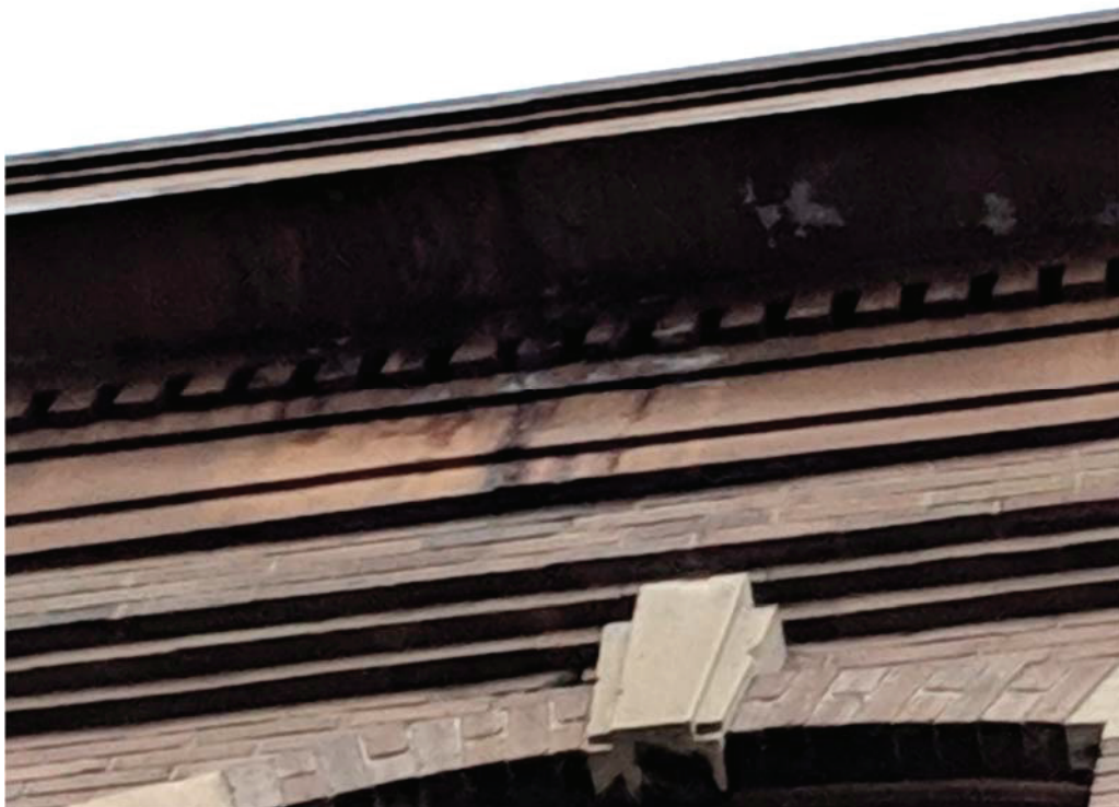
Photo 19: Corrosion and peeling on underside of cornice
