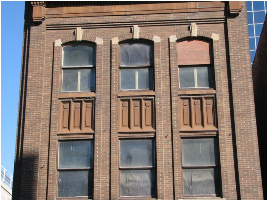
Metal spandrel panels separating first and second floor windows, 2010 (City of Regina)
