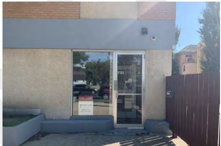
West door on north elevation, introduced when the main floor was reorganized to suit commercial use. Door is in fair condition.
