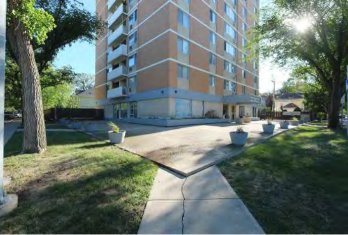
Looking toward northeast corner, showing cracked sidewalk and concrete pad elevated from sidewalk, causing an issue for accessibility.
