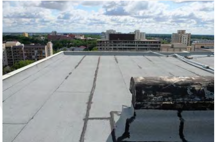
Roof looking east, showing patched roof where some water has infiltrated the roofing after a heavy rain.
