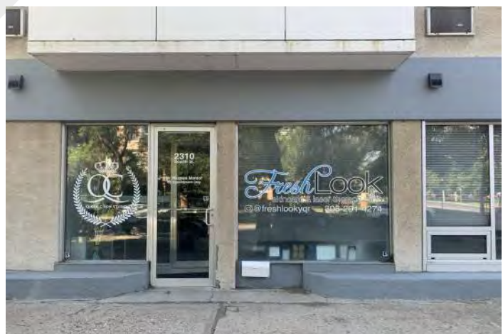
East elevation door for existing commercial space. Door to the north has been infilled with a larger window in a past intervention.
