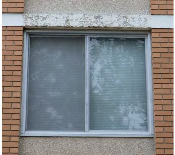
Detail of a window on the north elevation, showing built up caulking and deteriorating painted concrete slab edge.
