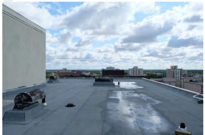
Roof looking east, showing water pooling on the south side. The roof slope should be revised for adequate drainage during the next roof replacement.
