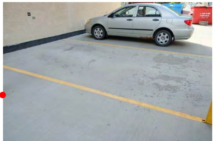
West concrete pad showing cracking and spalling. Concrete was poured in the last two years.
