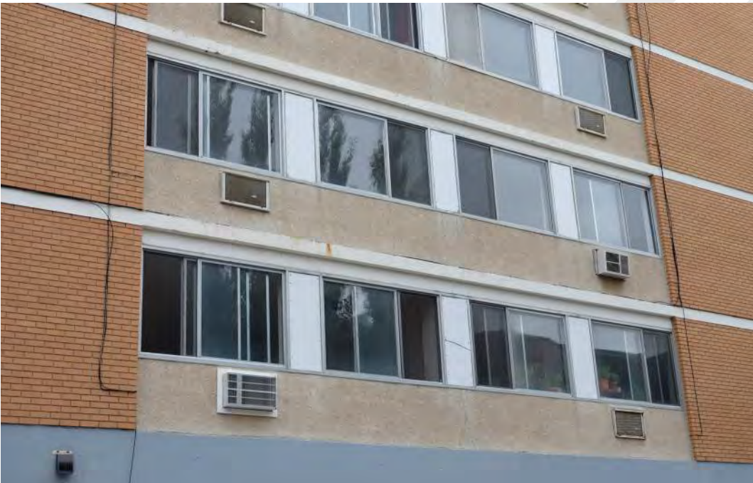
West façade, showing overall of aluminum windows in poor condition.
