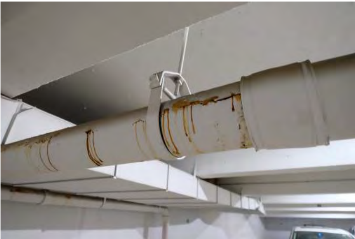
Water staining from leaking mechanical pipes.
