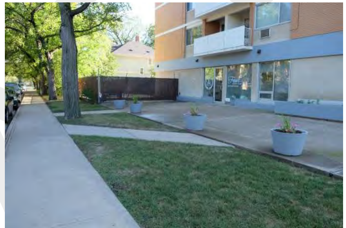
East Concrete pad and surrounding sidewalk. The concrete pad is elevated one to two inches from the sidewalk.
