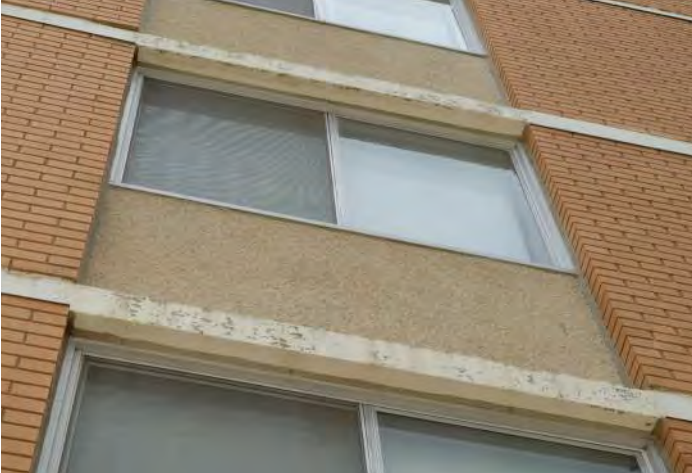
North façade, showing deteriorating concrete slab edge and excessively caulked aluminum windows.
