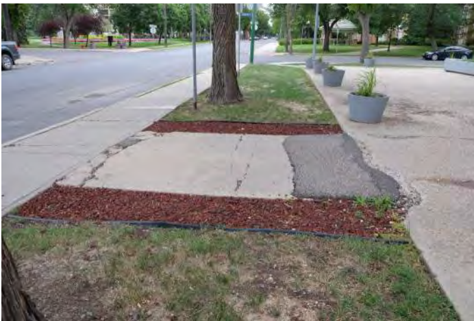
Concrete and red lava rock at north side of the site. Asphalt has been poured to ramp up from sidewalk level to concrete pad.
