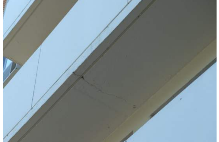
Detail of cracking down the centre of the third floor balcony.
