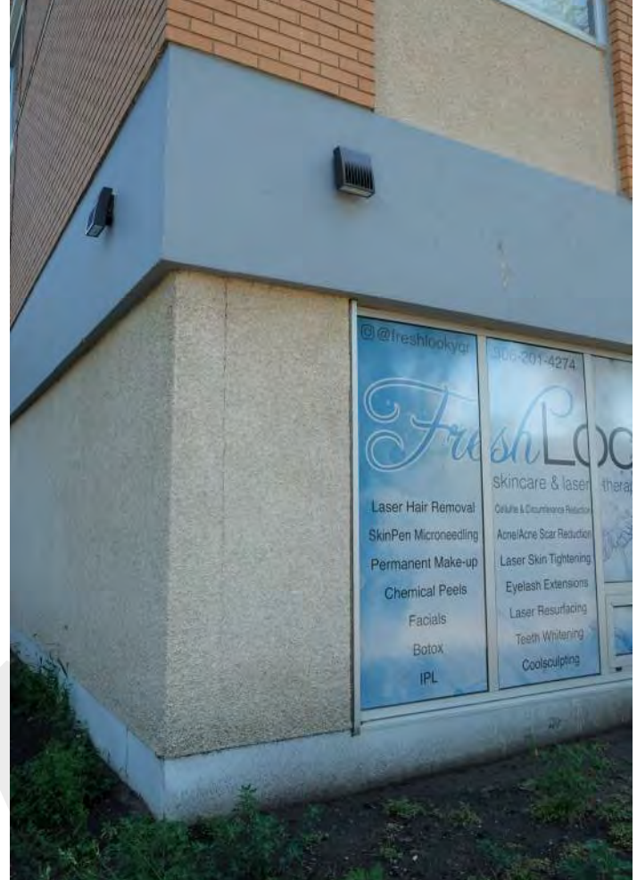
North façade, showing cracked stucco and hairline cracks in concrete
