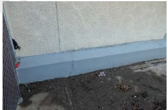
East façade, showing portion of cracked stucco and cracked concrete.
