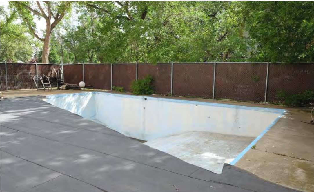
Southeast corner looking south, SBS covering on concrete patio surface to prevent water infiltration into the parking garage.
