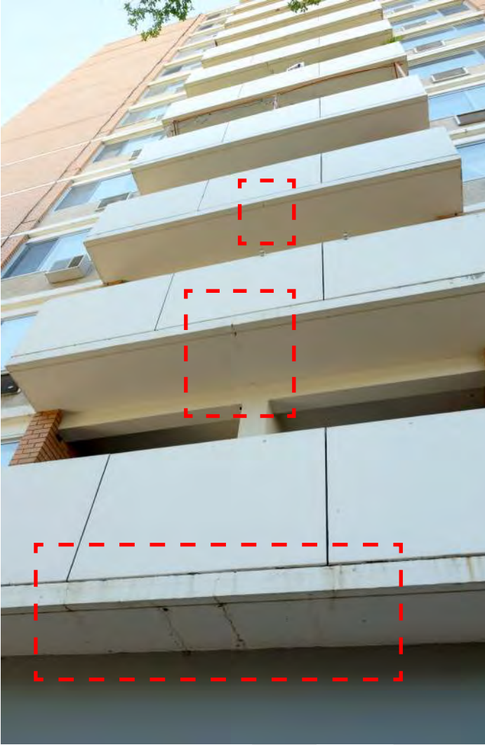
East façade, showing cracking down the centre of the majority of projecting balconies. Cracks are most severe on the second floor balcony.
