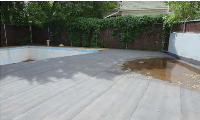
Southeast corner looking south, SBS covering on concrete patio surface to prevent water infiltration into the parking garage.
