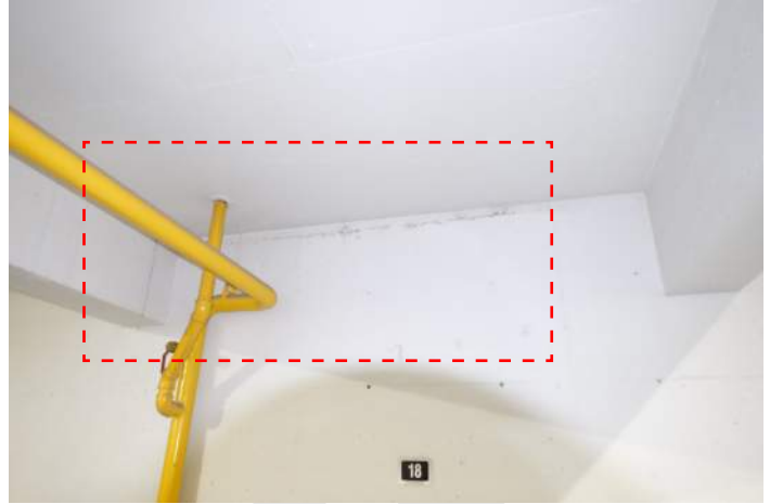
Crack and water staining on parkade wall.
