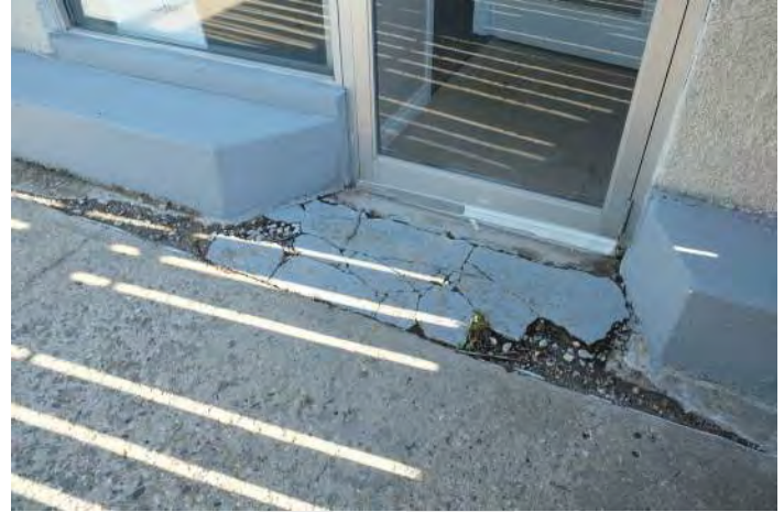
West corner of north façade, showing cracked concrete at door.
