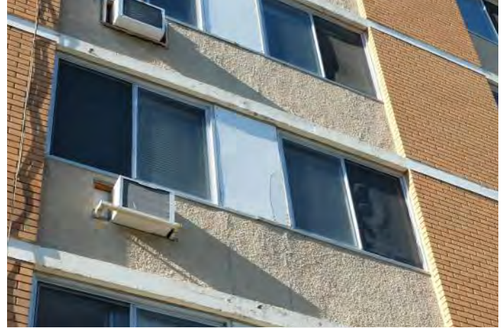
South elevation window detail. Showing excessively caulked window frames, cracked prefinished panel, and spalling concrete slab edge with peeling paint.
