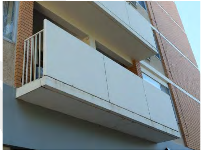
Detail of cracking down the centre of the second floor balcony. Also showing cracking and staining on the front face of the concrete slab.
