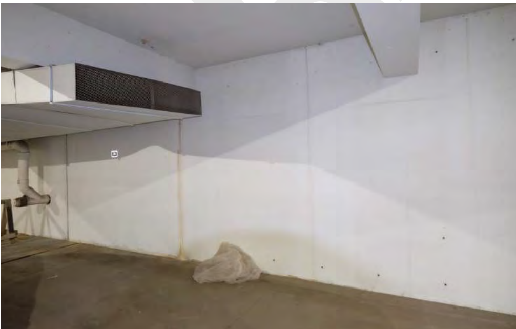
Water staining on west parkade wall.
