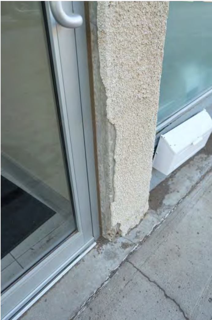
East façade, showing spalled and cracked stucco.
