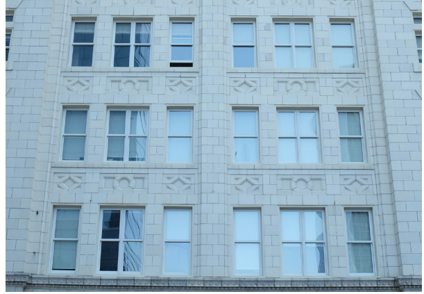
Figure 5.5.2 West elevation windows; levels 2-4. The majority of windows appear to be PVC (Polyvinyl Chloride) and should be replaced with wood windows when replacement is required.
