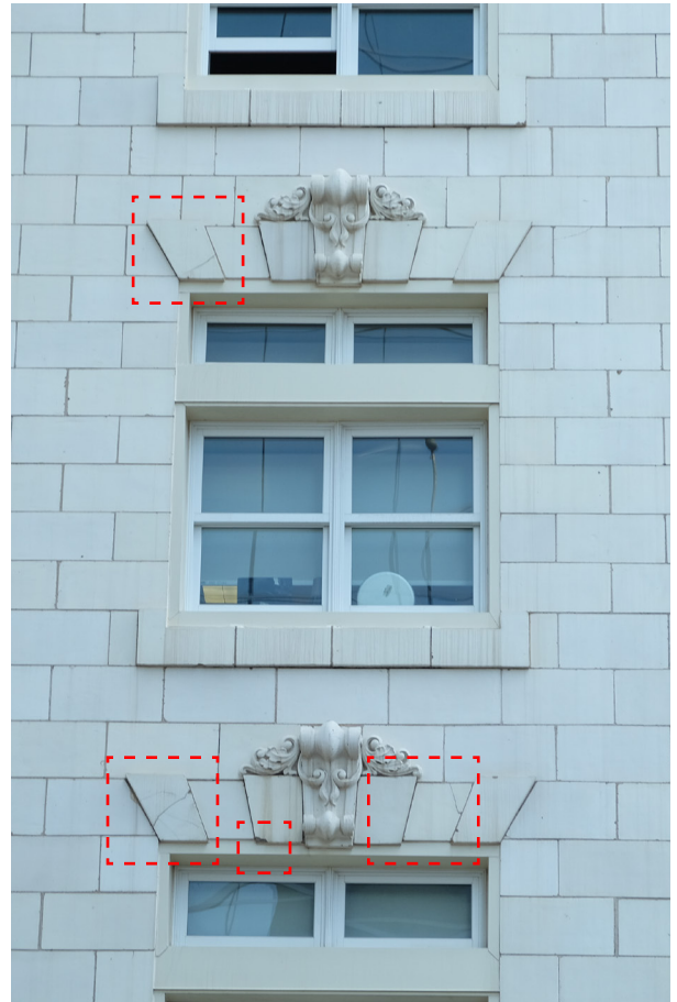
Figure 5.3.5 West terra cotta façade; outlining cracked and spalled terra cotta units
