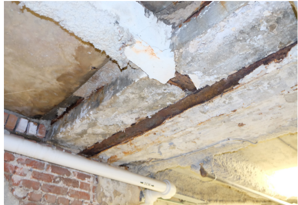
5.3.10 Concrete crumbling off of rusted steel beam
