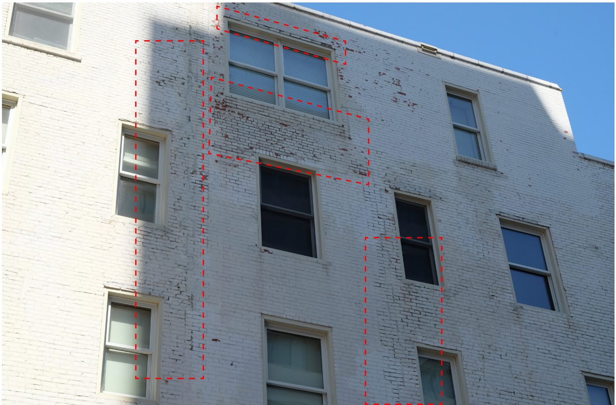
Figure 5.3.5 Mortar and brick cracking on south façade, particularly at the previously infilled portion (not limited to the areas outlines in red)
