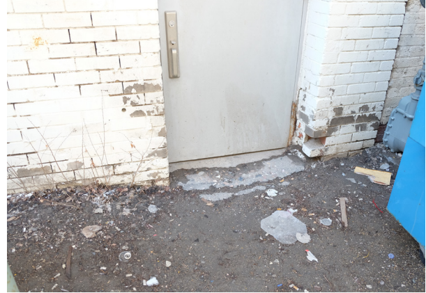
Figure 5.3.7 Discolouration and deterioration of brick masonry at the ground level.
