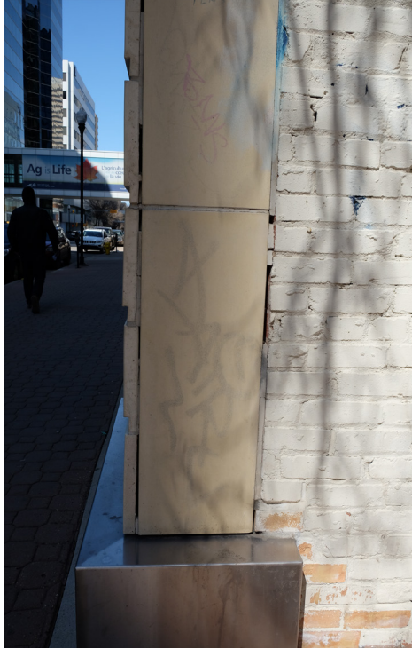
Figure 5.3.5 West terra cotta façade; outlining cracked and spalled terra cotta units
