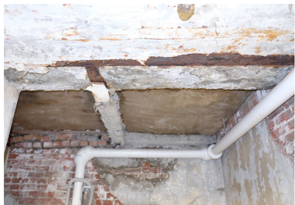
Figure 5.3.13 Loose bricks at foundation wall (looking west), discolouration and deterioration due to water infiltration.
