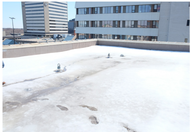
Figure 5.4.3 West SBS Modified Bitumen Roofing System
