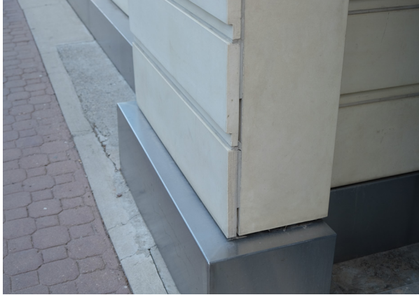
Figure 5.3.1 Mortar missing in numerous masonry unit joints
