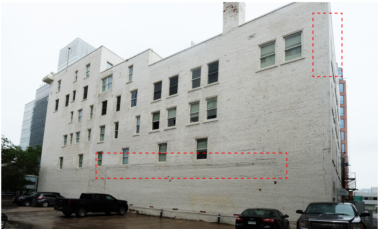
Figure 5.3.8 South brick façade, outlining areas of the façade where brick staggers vertically. Brick above windows at the southeast corner appears to be bowing and pulling away from the structure (right dashed outline)
