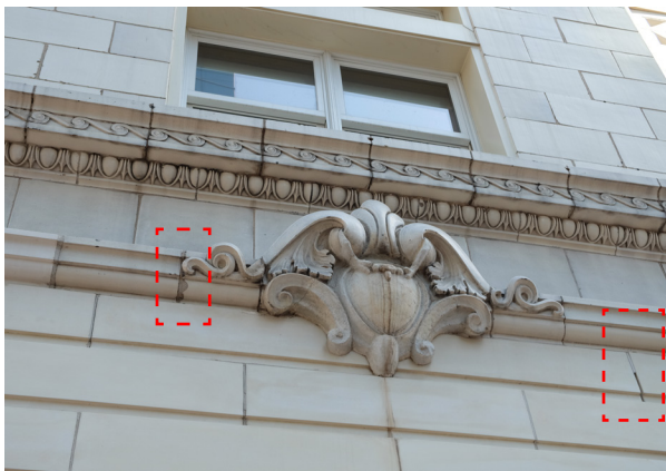
Figure 5.3.4 West terra cotta façade; outlining spalling, stained masonry, gaps and cracks in mortar
