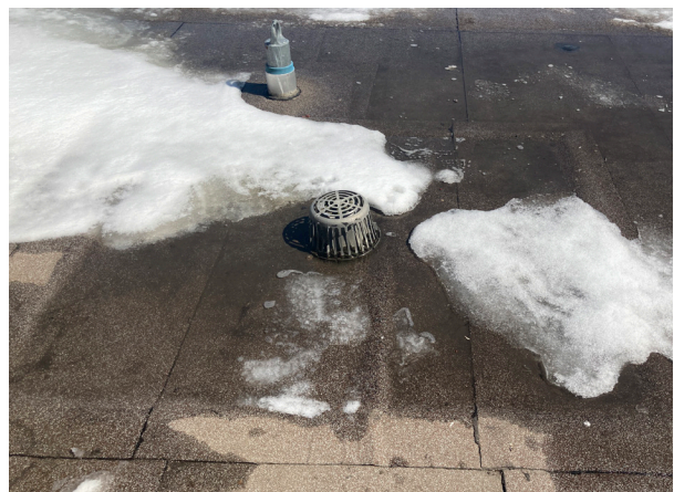
Figure 5.4.5 Roof drain is not located in the center of the roof which makes drainage less efficient. Ponding appears like it might be possible with ridges noticed in the top layer of the roofing.
