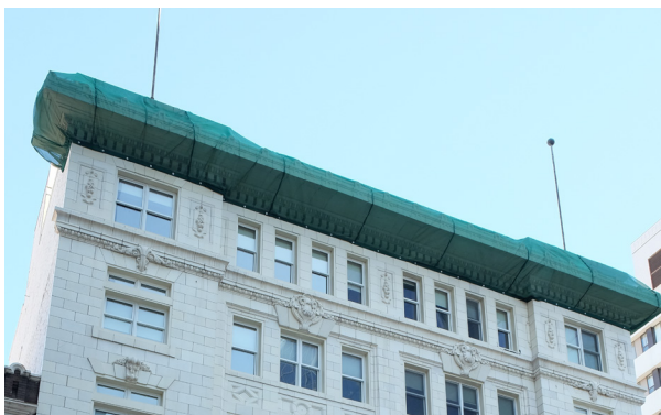
Figure 5.4.6 Cornice has been wrapped in netting as a preventative measure
