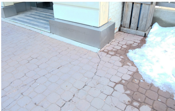
Figure 5.3.9 Cracking sidewalk at southwest entrance.
