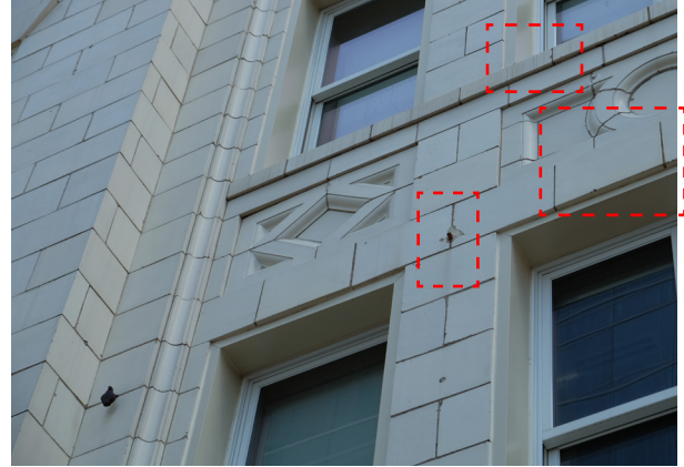
Figure 5.3.2 West terra cotta façade; outlining spalled and chipped terra cotta units.
