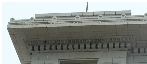
Figure 5.4.1 Ornamented cornice showing signs of water penetration
