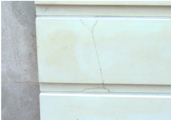
Figure 5.3.3 Cracked masonry unit to be repaired or replaced.
