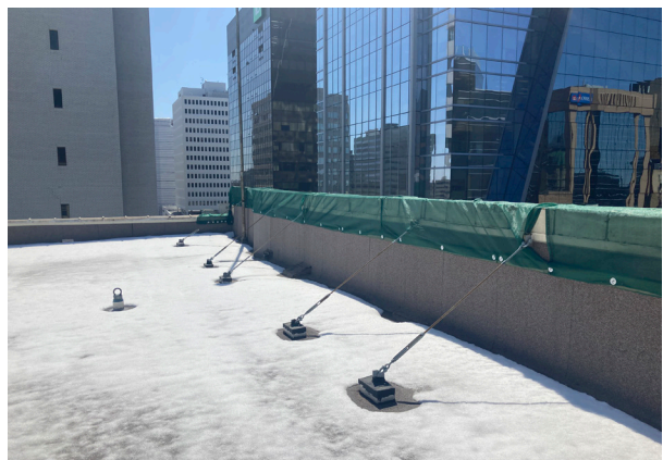
Figure 5.4.7 West parapet anchored onto roof
