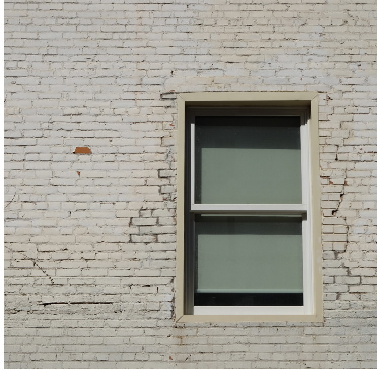
Figure 5.3.5 West terra cotta façade; outlining cracked and spalled terra cotta units
