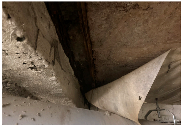
Figure 5.3.12 Membrane has peeled off of concrete slab, rusted steel beam exposed
