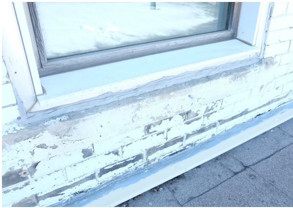
Figure 5.5.3 Some joints at the window sills on the upper east façade have been caulked over. Could mean that window replacement is required.
