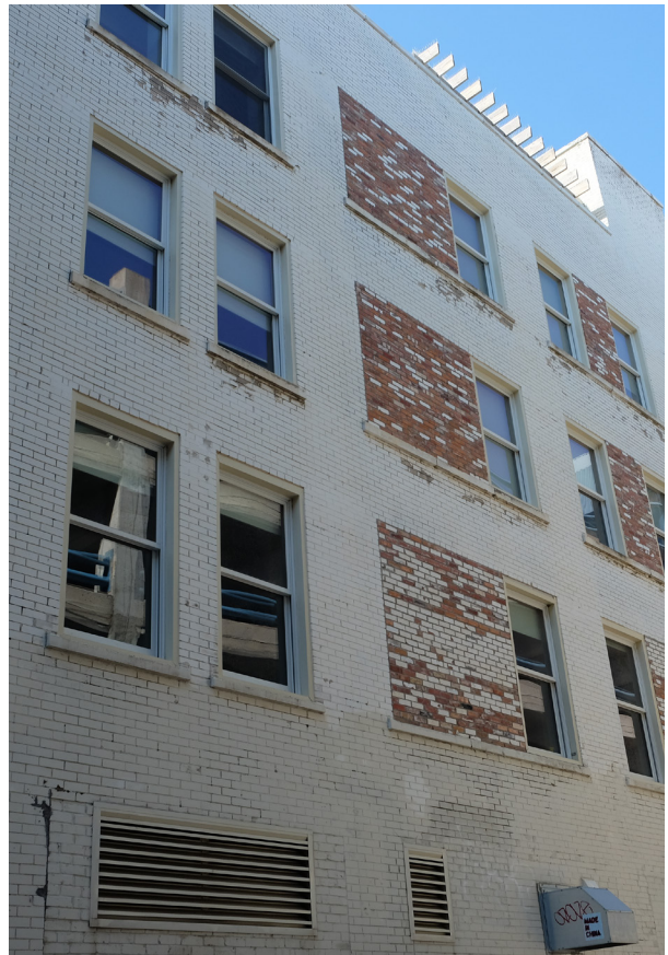
Figure 5.5.5 Potential water infiltration at the east elevation windows is evident from the discolouration at the concrete window sills.
