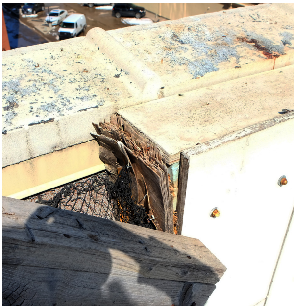
Figure 5.4.4 Wall construction of the interior face of the parapet on the east side of the building
