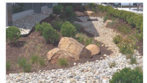
Water management by drainage channel and catch basin
