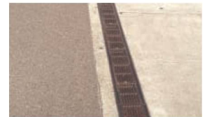
Water management by trench drain
