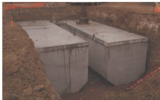
Rainwater Harvesting Cistern
