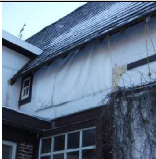
Water proofing installed over stucco at back due to suspected moisture transfer
