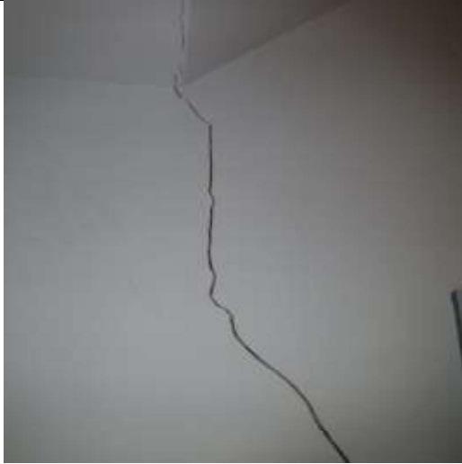
Large cracking in main floor stairwell
