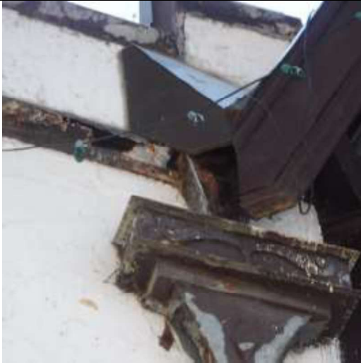
Rusted/damaged/leaking flashings, gutters, downspouts
