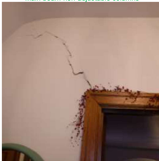
Cracking in walls/ceilings from pressure and settlement
