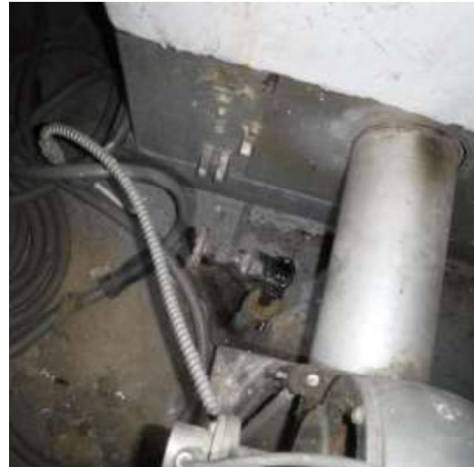
Leaking oil line near boiler
