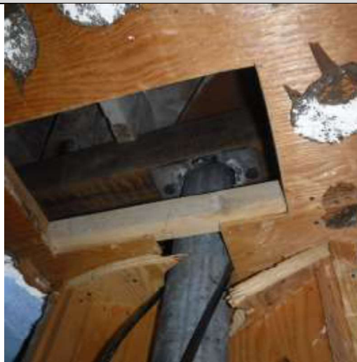
Main beam-non-adjustable columns
