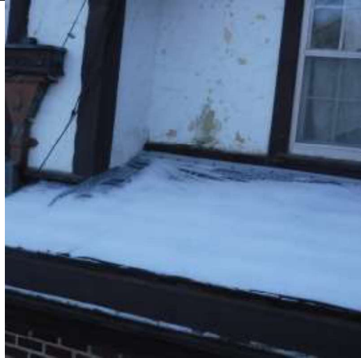
Suspected leaking flashing at back lower roof-interior damage
