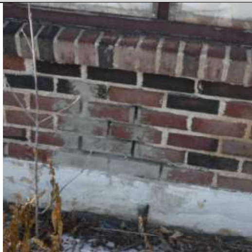
Cracking in brick and stucco
