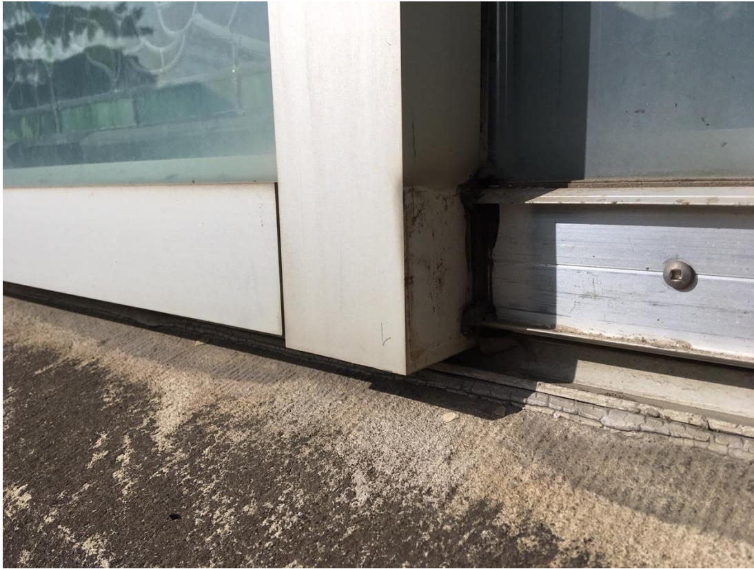
Air gap between aluminum window frame and stone
