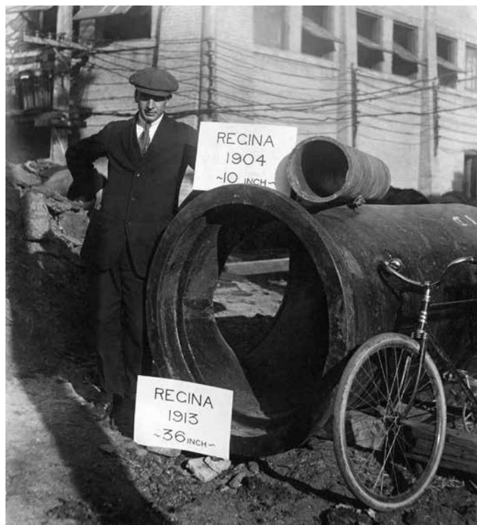
A man standing beside different sizes of pipes used to supply the city with water from Boggy Creek, 1913. (City of Regina Archives CORA-RPL-B-0386)
