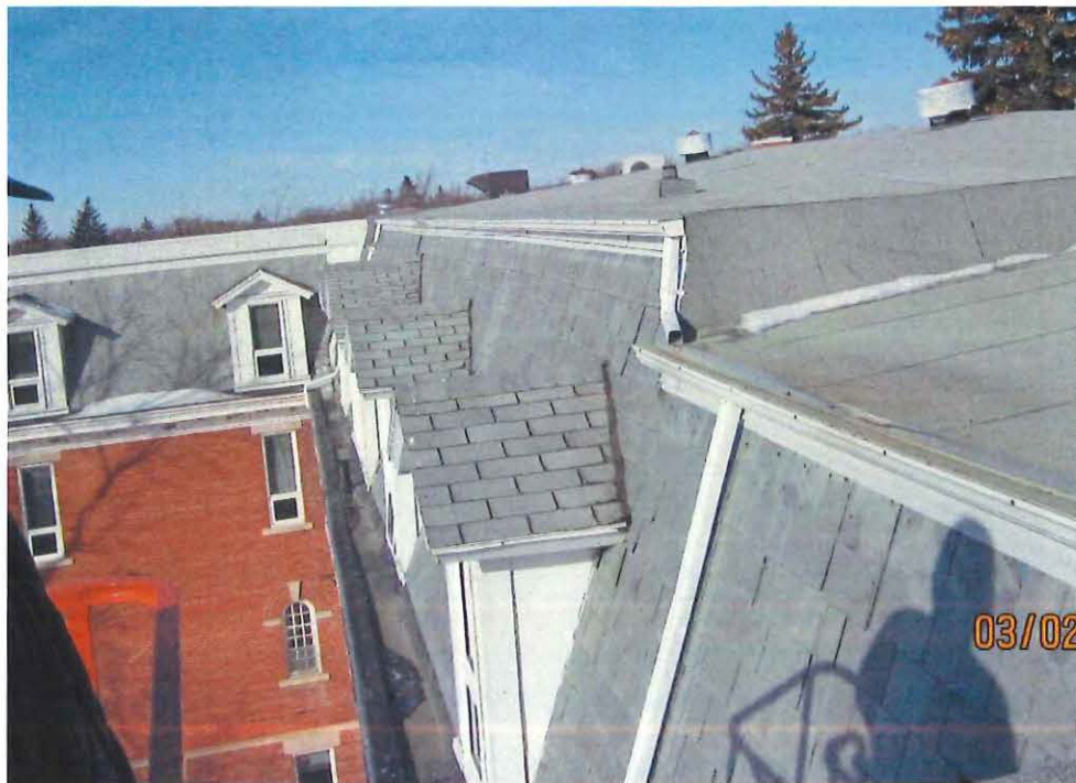
Figure 40 – South façade – roof caulk at dormers; missing top row of slates (note asphalt shingles on dormers and no metal flashing)
