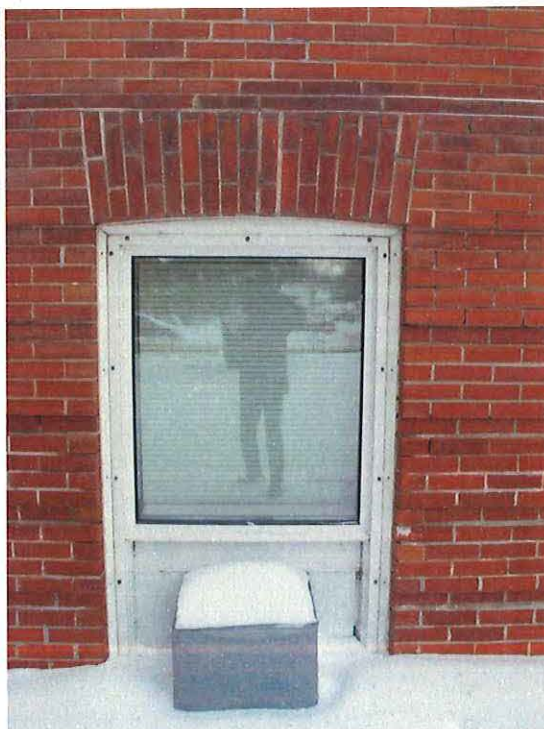
Figure 10 — remaining brick arch lintel on 1909 portion
