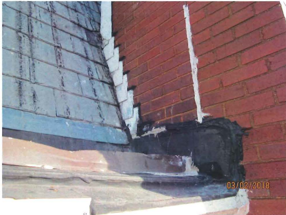
Figure 36 – top side of cornice with EPDM roofing and roof patch material at chimney
