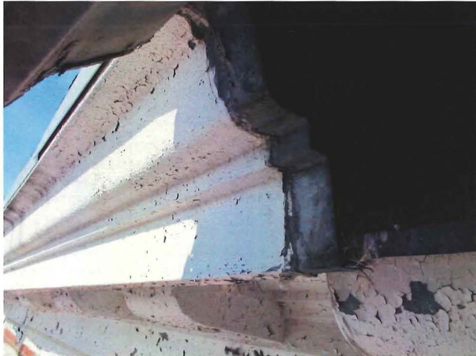
Figure 32 – profilled metal cornice on south face – showing profile at join
