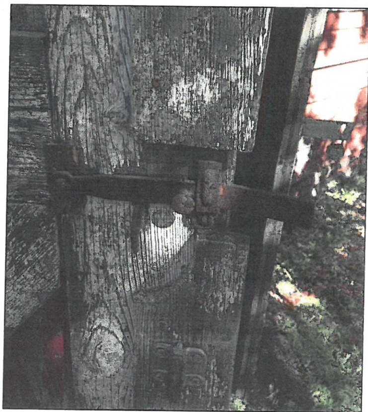
Figure 5. A close-up photo of the original door catch on the east carriage door.
