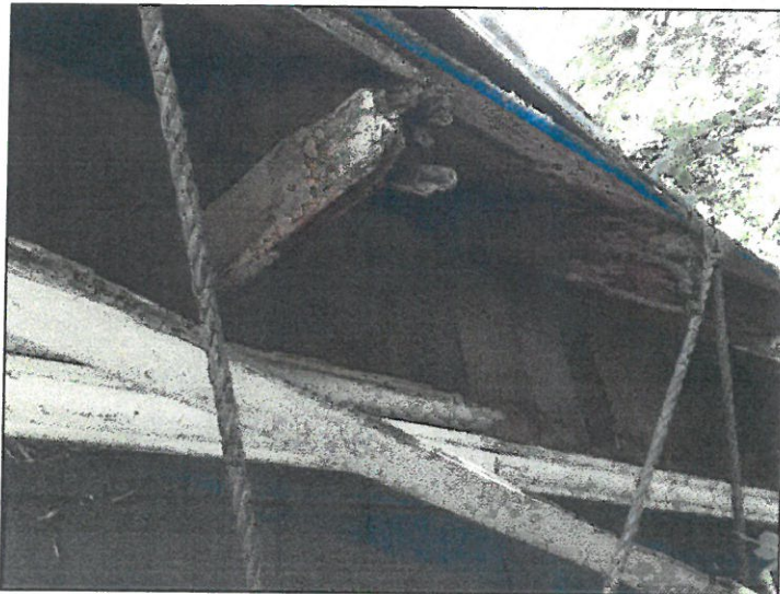
Figure 13. A close-up photo of the underside of the first floor roof overhang showing missing fascia and some soffit boards and rotted rafter tails.
