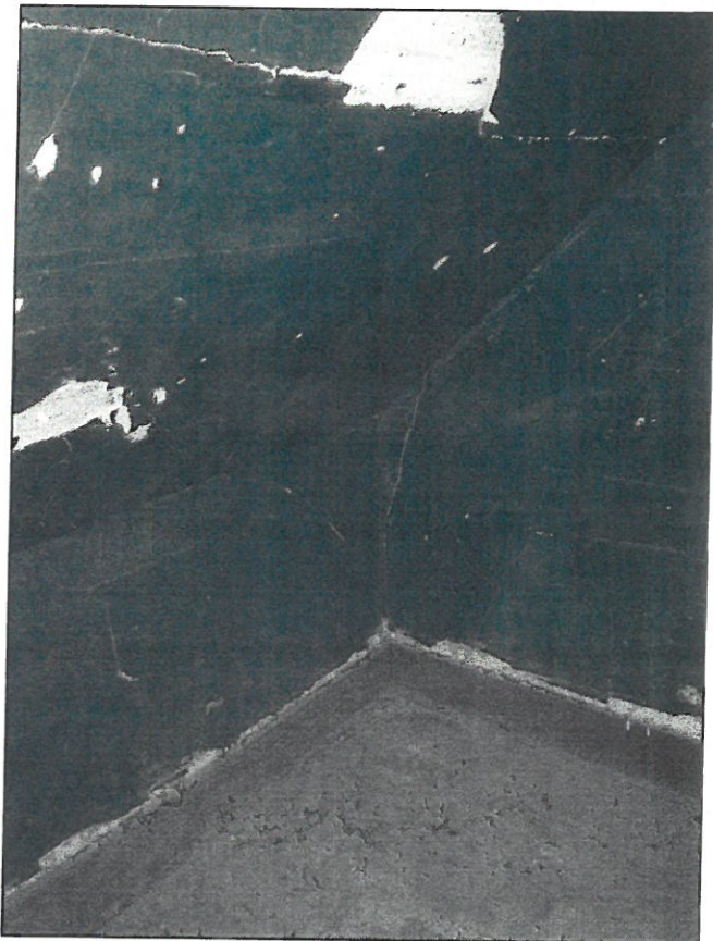
Figure 29. The second floor "carriage boy's" apartment. The lath and plaster walls and ceiling were in a bad state of repair. The vertical grain tongue and groove wood floor is visible with fir baseboards.
