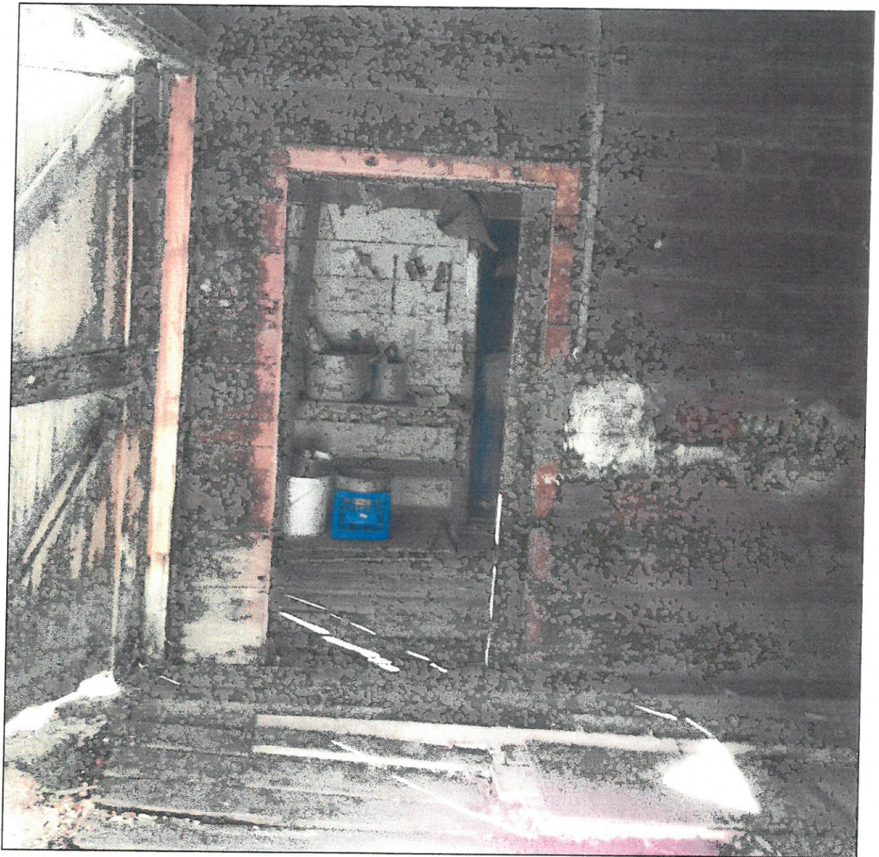
Figure 25. An interior view within the central carriage housing portion of the building, looking west through a sliding pocket door into the anteroom of the animal housing and feed storage areas. The poor condition of the doors and floor are evident. The fir boards lining the interior walls were in good condition, however the floor boards were severely rotted.
