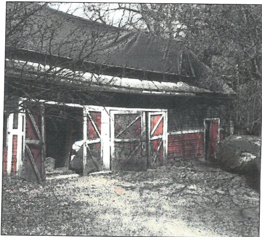
Figure 3. The south view of the carriage house. The two upper dormers are covered by a tarp to prevent further deterioration due to roof leakage. The two double carriage doors and the ice house door (far right) show evidence of the loss of structural integrity on this side of the building, necessitating a foundation replacement. Not visible in this photo is the walk in door to the animal housing area to the left.
