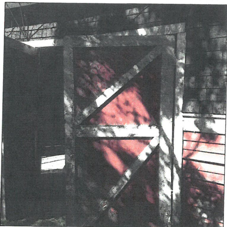
Figure 4. A close-up photo of the east carriage door. This door and the adjacent door to the immediate west are replacements from the original as they are constructed of plywood. As far as can be discerned, the pattern on the doors is likely original.
