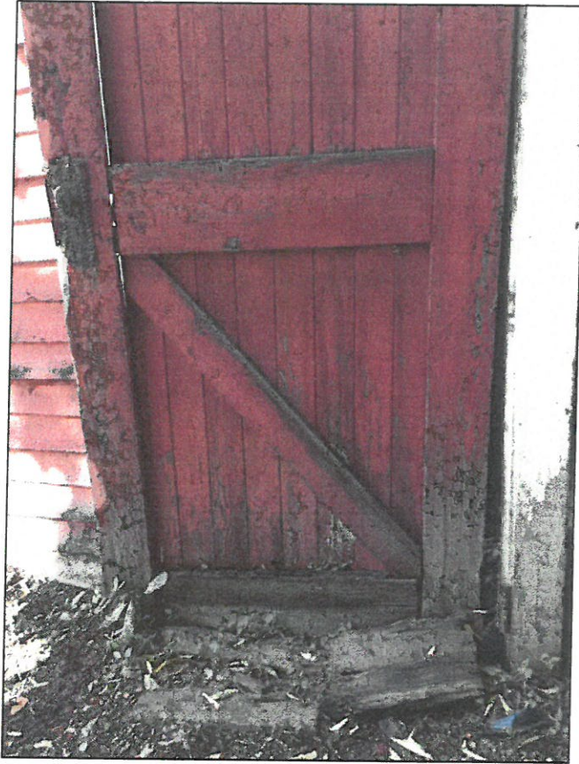
Figure 9. The east walk in door on the south side. This door accessed the ice house. Evidence of deterioration of this door is present. This door is a good example of the design model for exterior doors that need replacement.
