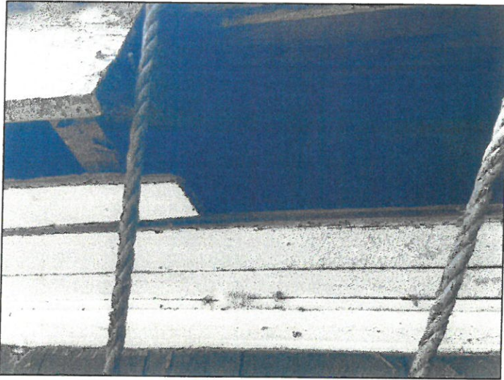
Figure 12. A close-up photo of the underside of the first floor roof overhang showing missing fascia and some soffit boards.
