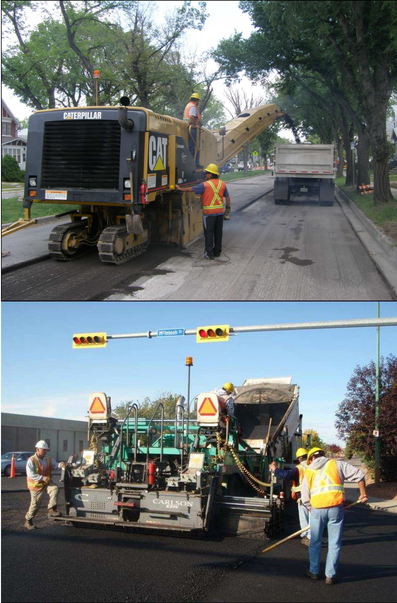
City Crews Milling and Paving as part of Street Infrastructure Renewal Program
