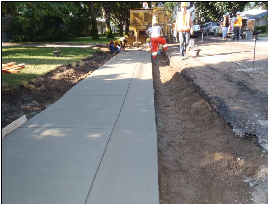
Slip Forming New Sidewalk as part of LIP Project
