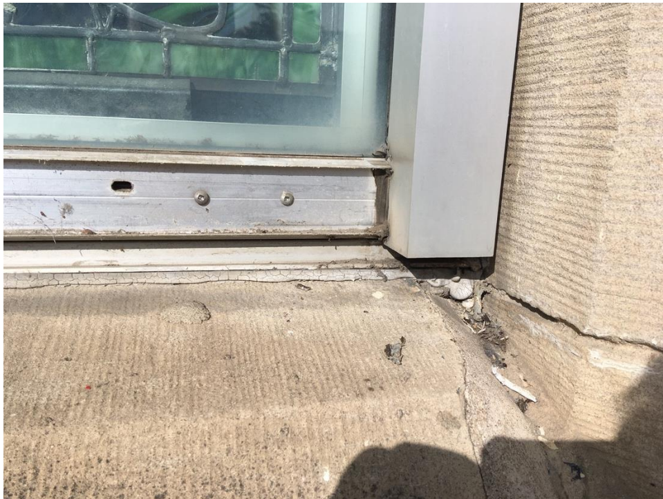
Detail of Aluminum Cap and Pressure Plate
