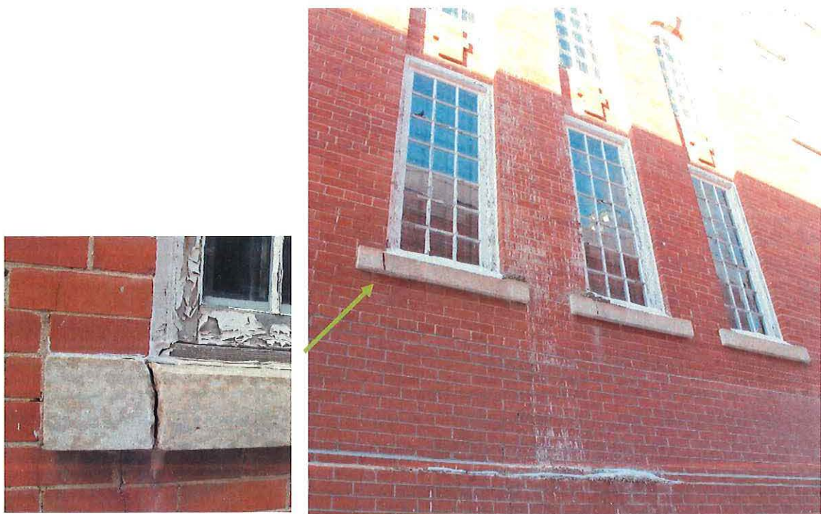
Figure 29 – South face of Chapel showing cracked Tyndall Stone sills on two windows
