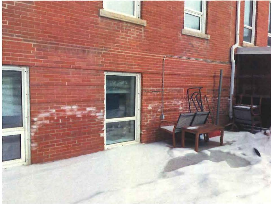
Figure 20 – South façade where wicking up of moisture is evidenced by the efflorescence on the bricks
