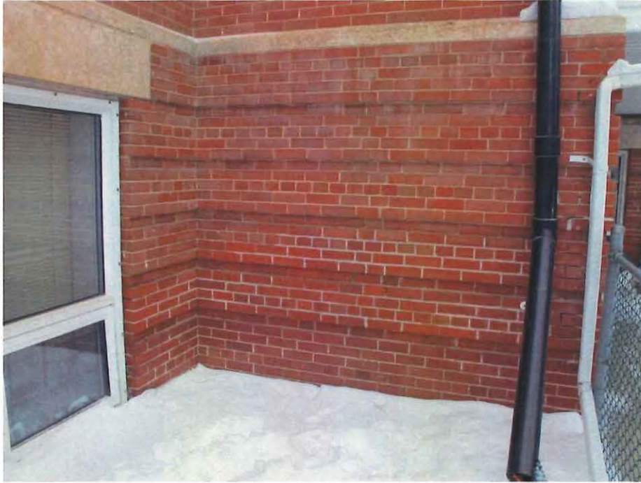
Figure 18 – Southwest corner of West façade – areas where more deterioration was noticed
