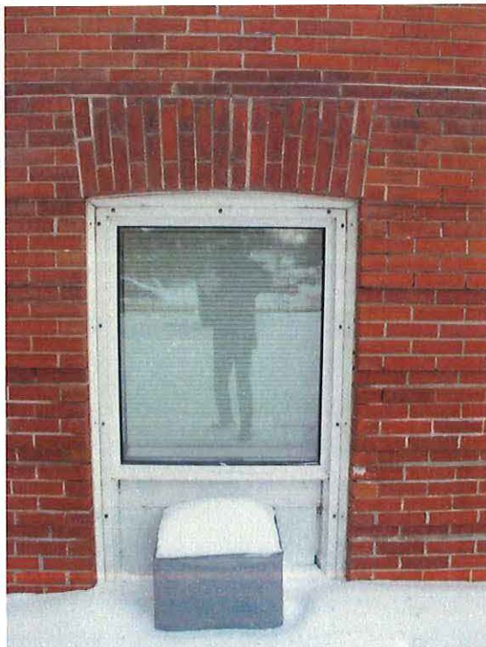
Figure 10 – remaining brick arch lintel on 1909 portion
