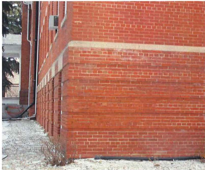
Figure 7 – Rusticated brick masonry on the 1924 portion with sloped Tyndall Stone belt course
