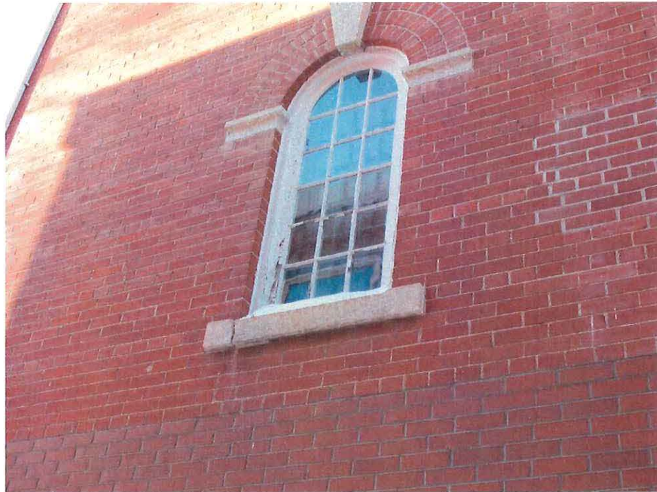
Figure 28 – South face of Chapel showing severely cracked Tyndall Stone sill
