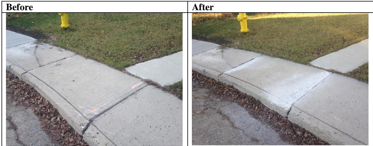
**Concrete Replacement:** This method is used to repair sidewalk deficiencies that are too severe for other treatments by replacing individual or multiple panels of sidewalk. This process involves the removal of the existing poor segments and pouring a new sidewalk. (\$540.00 per square meter, pedestrian ramps \$580 per square meter)
