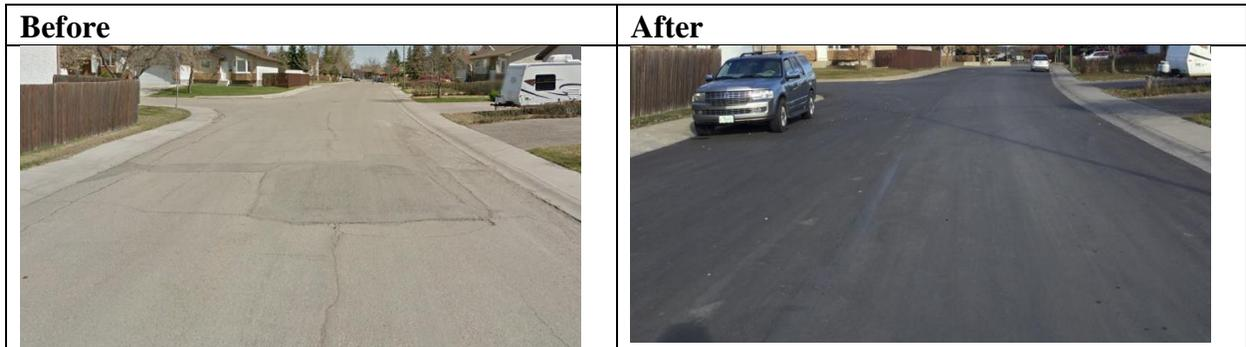
**Rehabilitation:** This is generally a thicker layer of asphalt (average 50 mm) placed on a milled surface of existing asphalt after milling and tack coat has been applied. Rehabilitation paving is best suited when pavement is in fair condition and concrete is in poor to fair condition. Rehabilitation is at least 10 years or more between cycles so minimal concrete and sewer work is completed as part of the repairs. (~\$235 per linear meter of road)
