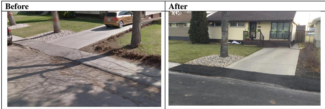
**Catch Basin Repair:** When the top of the catch basin is caving in or heaving, it can be adjusted or rebuilt in order to bring it into alignment with the road surface and improve drainage and driving conditions. (Adjustment \$1,000, rebuild \$3,300)
