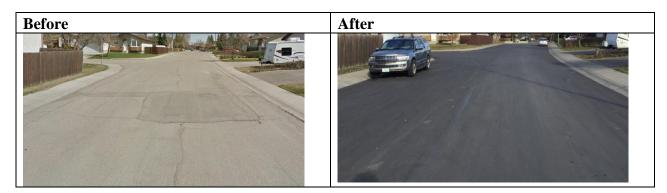
**Rehabilitation:** This is generally a thicker layer of asphalt (average 50 mm) placed on a milled surface of existing asphalt after milling and tack coat has been applied. Rehabilitation paving is best suited when pavement is in fair condition and concrete is in poor to fair condition. Rehabilitation is at least 10 years or more between cycles so minimal concrete and sewer work is completed as part of the repairs. (~\$235 per linear meter of road)
