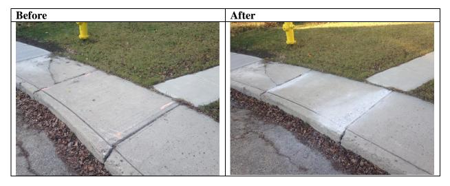
**Concrete Replacement:** This method is used to repair sidewalk deficiencies that are too severe for other treatments by replacing individual or multiple panels of sidewalk. This process involves the removal of the existing poor segments and pouring a new sidewalk. (\$540.00 per square meter, pedestrian ramps \$580 per square meter)
