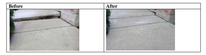
**Asphalt capping:** is a low cost option involving the placement of an asphalt overlay on a sidewalk that requires immediate attention due to severe sidewalk deficiencies. This method can be used to quickly address trip hazards and provide a smooth walking surface. It can also address concrete deficiencies on sidewalks that have no gutter or are separate from the gutter, which cannot be mudjacked. (\$53 per linear meter)
