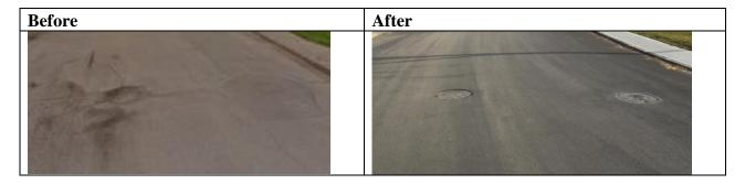
**Thin Lift:** This is the application of a thin layer of asphalt (average 40 mm) placed either directly over existing asphalt or has had minimal milling done in advance of the application of new asphalt. Thin lift paving is best suited when pavement is in fair to good condition, minimal drainage issues exist, concrete is in fair to good condition. (~\$195 per linear meter of road)
