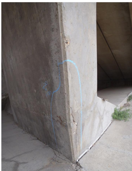
Typical delamination/spalling at pier.
