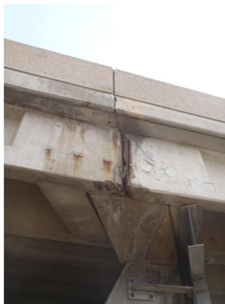
Typical spalling/corrosion of girder reinforcing steel at pier.
