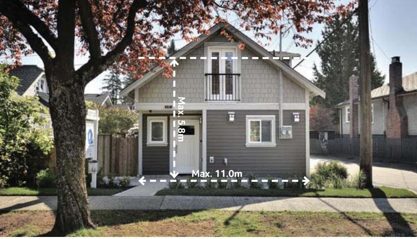
The width of exterior building walls for Laneway and Garden Suites should be determined based on applicable side yard setback requirements (Smallworks Studio).
