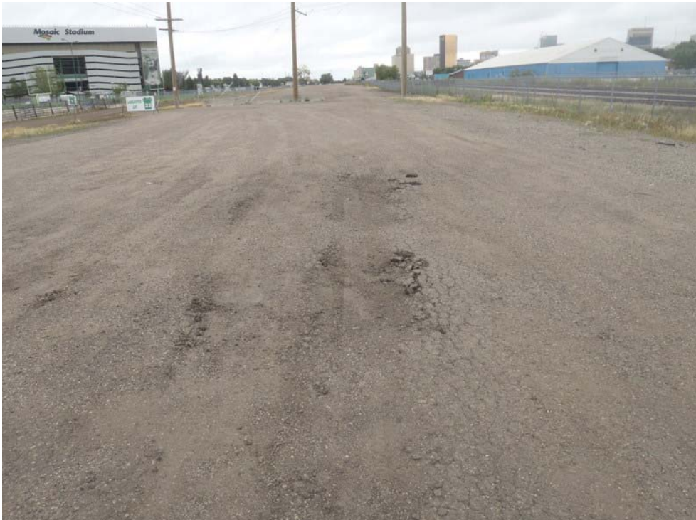
Photograph 6 – The Site appears to have been paved at one point; however, the asphalt is crumbling, and the Site is mostly gravel.
